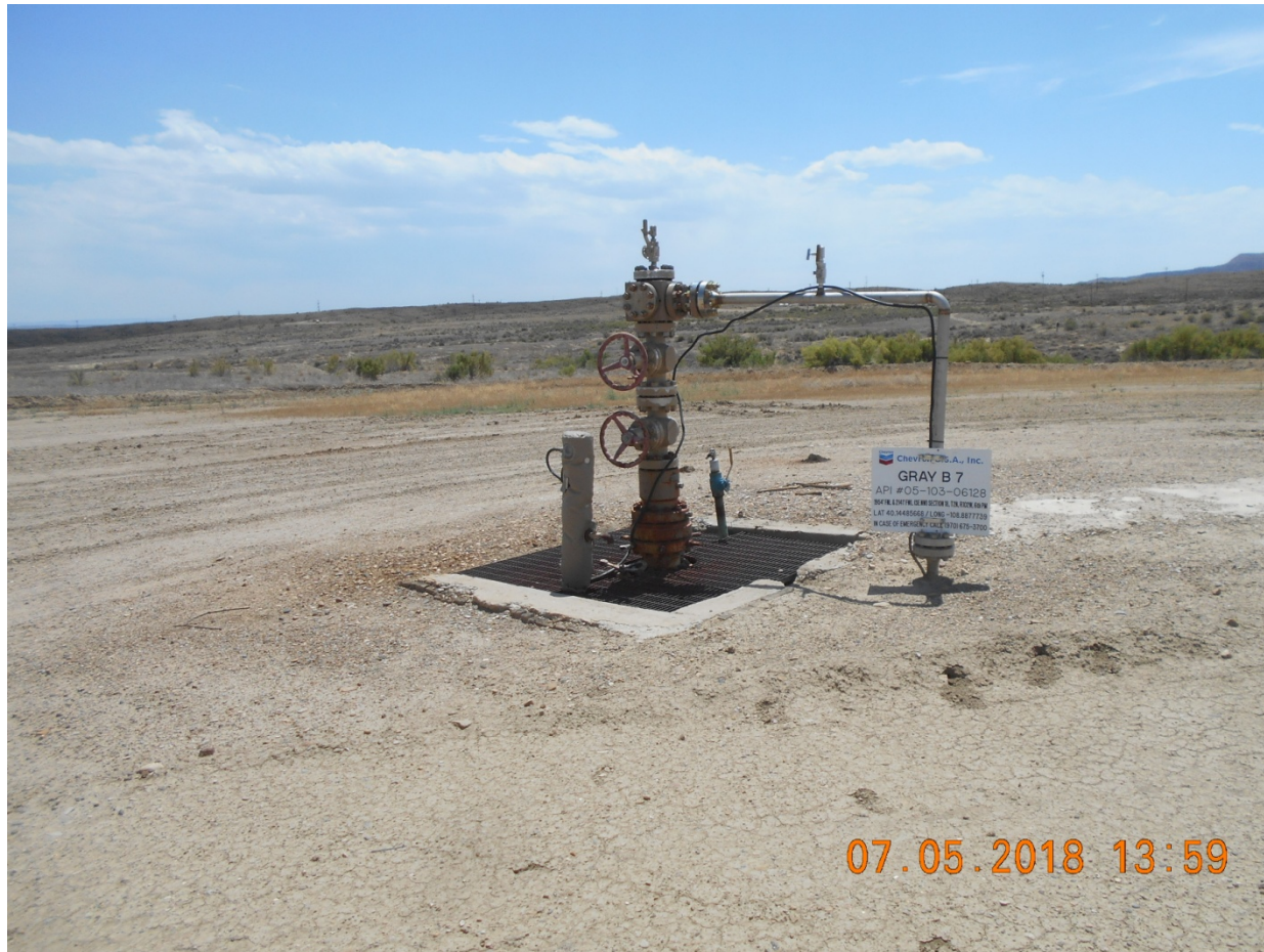
Injection Wellhead
