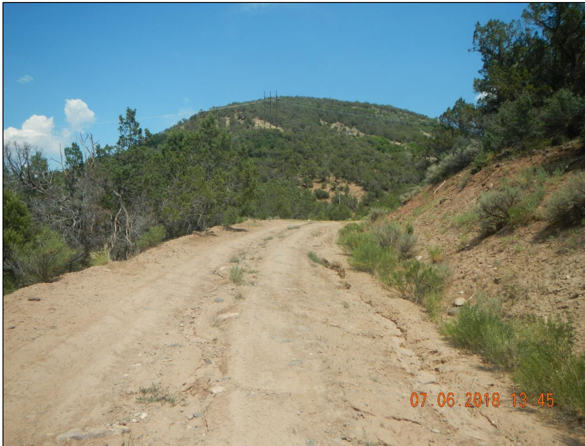
Ruts on access road are washing and moving sediment.
