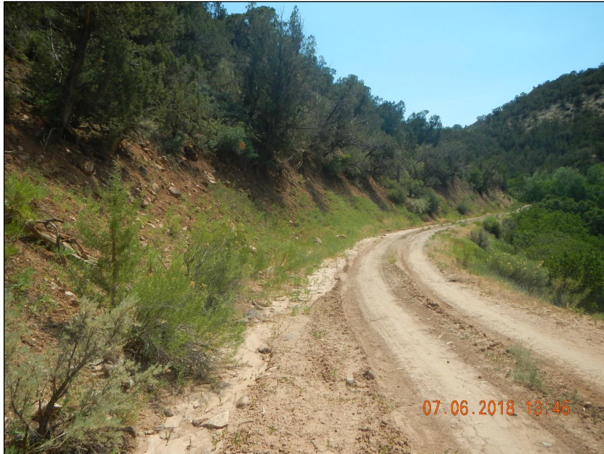
Sediment build up in road ditch.
