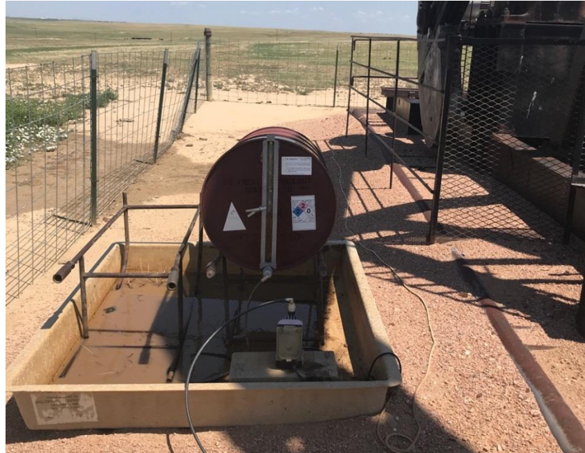
Photo#9 Chemical pump and tank
