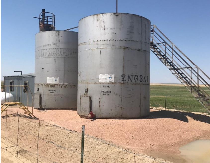
Photo#3 Produced water tanks
