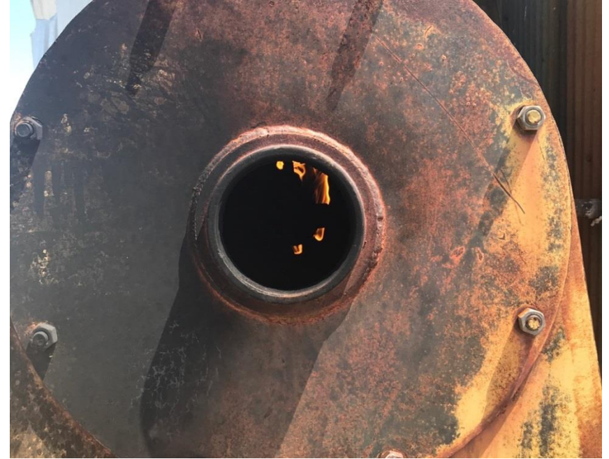
Photo#4 Burner stack missing sight glass or plug
