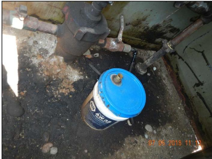
**Photo 3. Stained soil at wellhead. Lube oil stored without secondary containment.**
