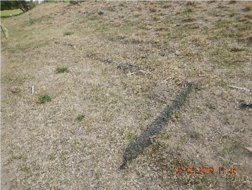
Photo 13: Deteriorated waddles and material netting.
