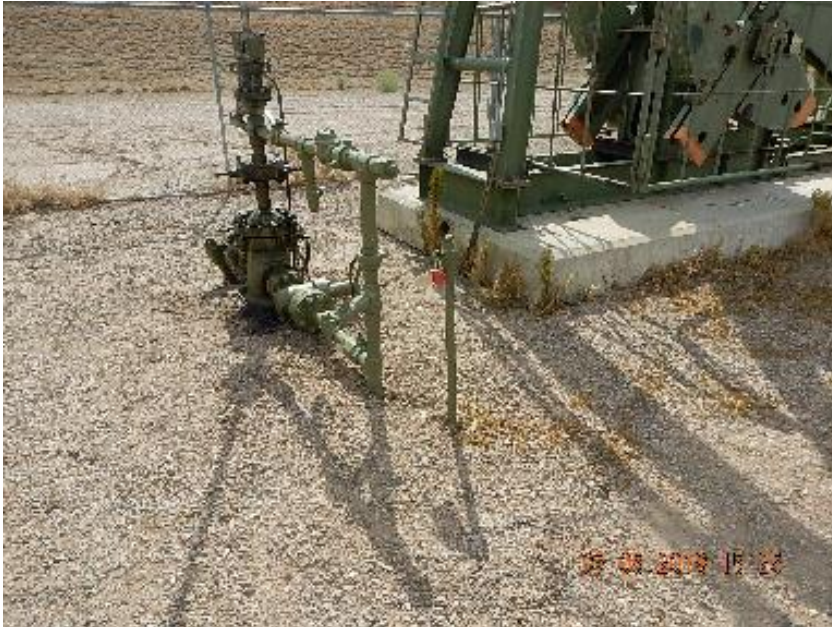
Photo 5: Unused riser at #4-1 wellhead.
