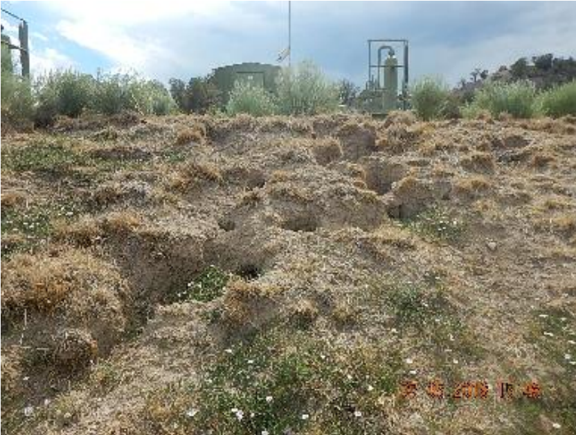
Photo 11: Erosion on NE corner looking up fill slope.
