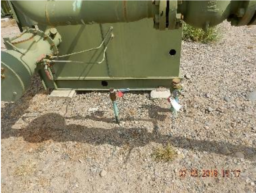
Photo 3: Unused riser at #4-3 separator.
