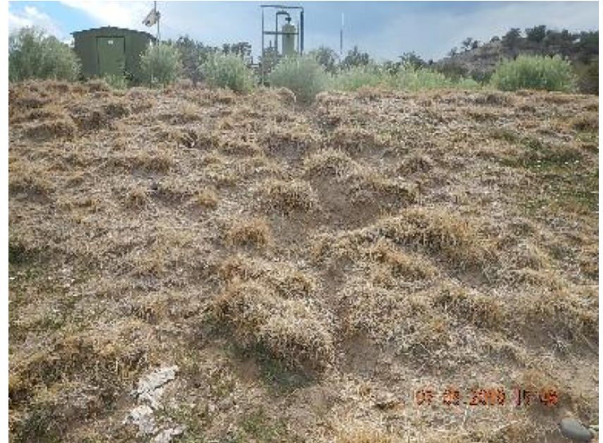
Photo 12: Erosion channel on fill slope.
