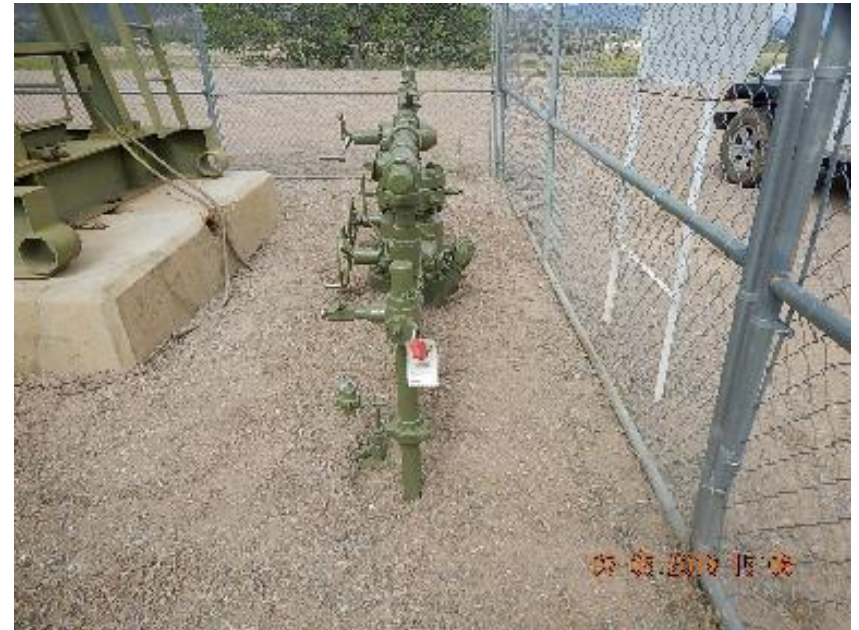
Photo 2: Unused riser at #4-3 wellhead.
