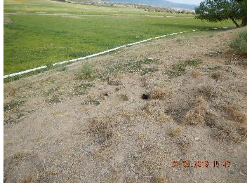
Photo 14: Animal burrows and erosion on E fill slope..
