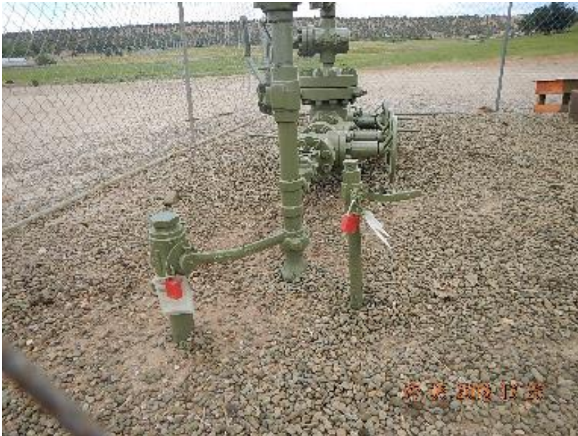
Photo 5: Unused risers at #5-3 wellhead.
