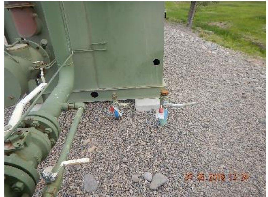
Photo 6: Unused risers at #5-3 separator.
