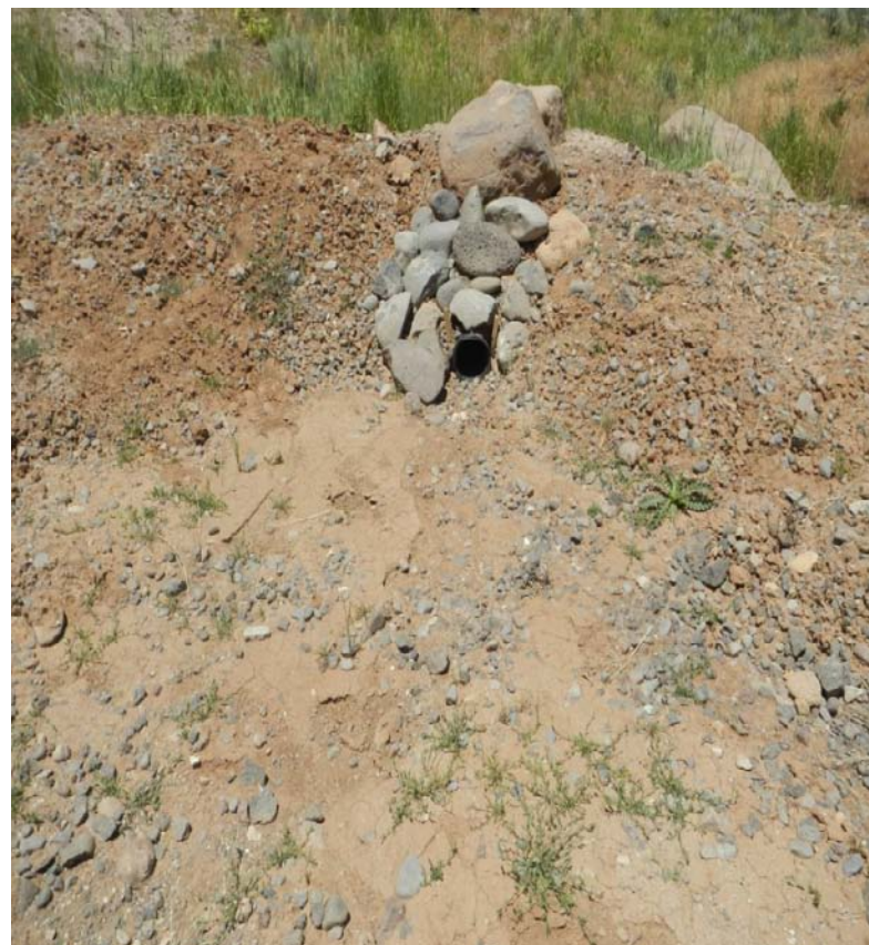
Photo#6: One Sediment trap is full to drain out level.
