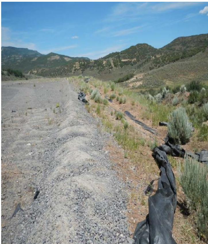
Photo#5: Liner has become debris
