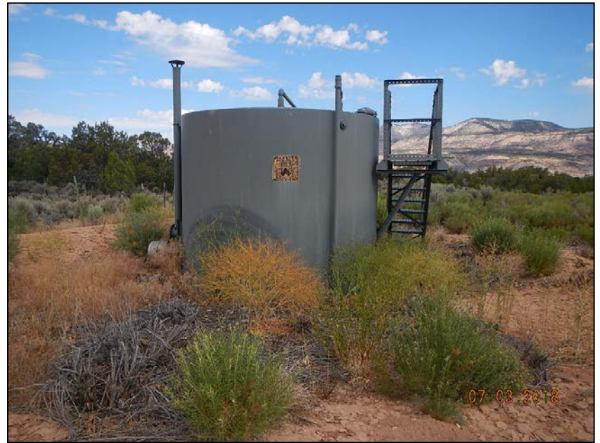
Photo 2. Tank label illegible and vegetation and debris in containment.
