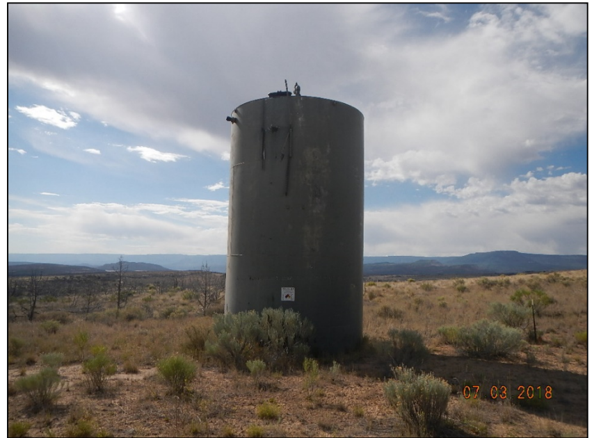
Photo 2. Tank scheduled for removal.
