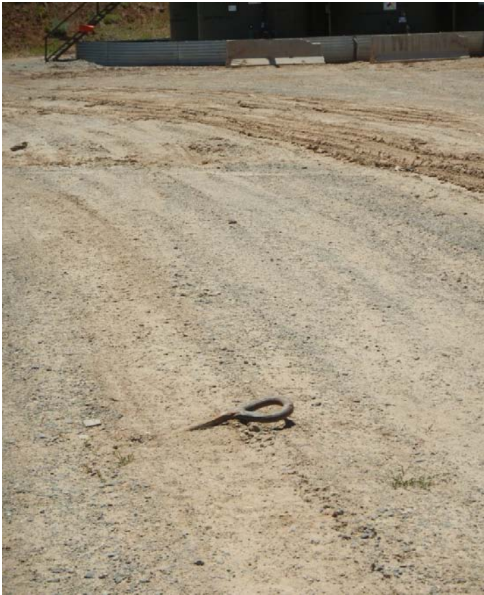
Photo#3: Two anchors noted run over & not marked..
