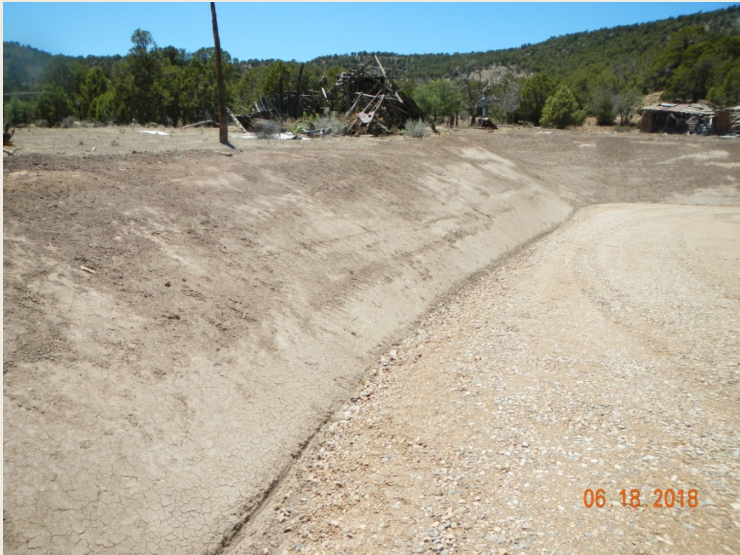
Photo 2. View of the southern portion of the project area from the southeastern corner facing westward. Run-on controls and stabilization measures are needed on these slopes until revegetation is achieved.
