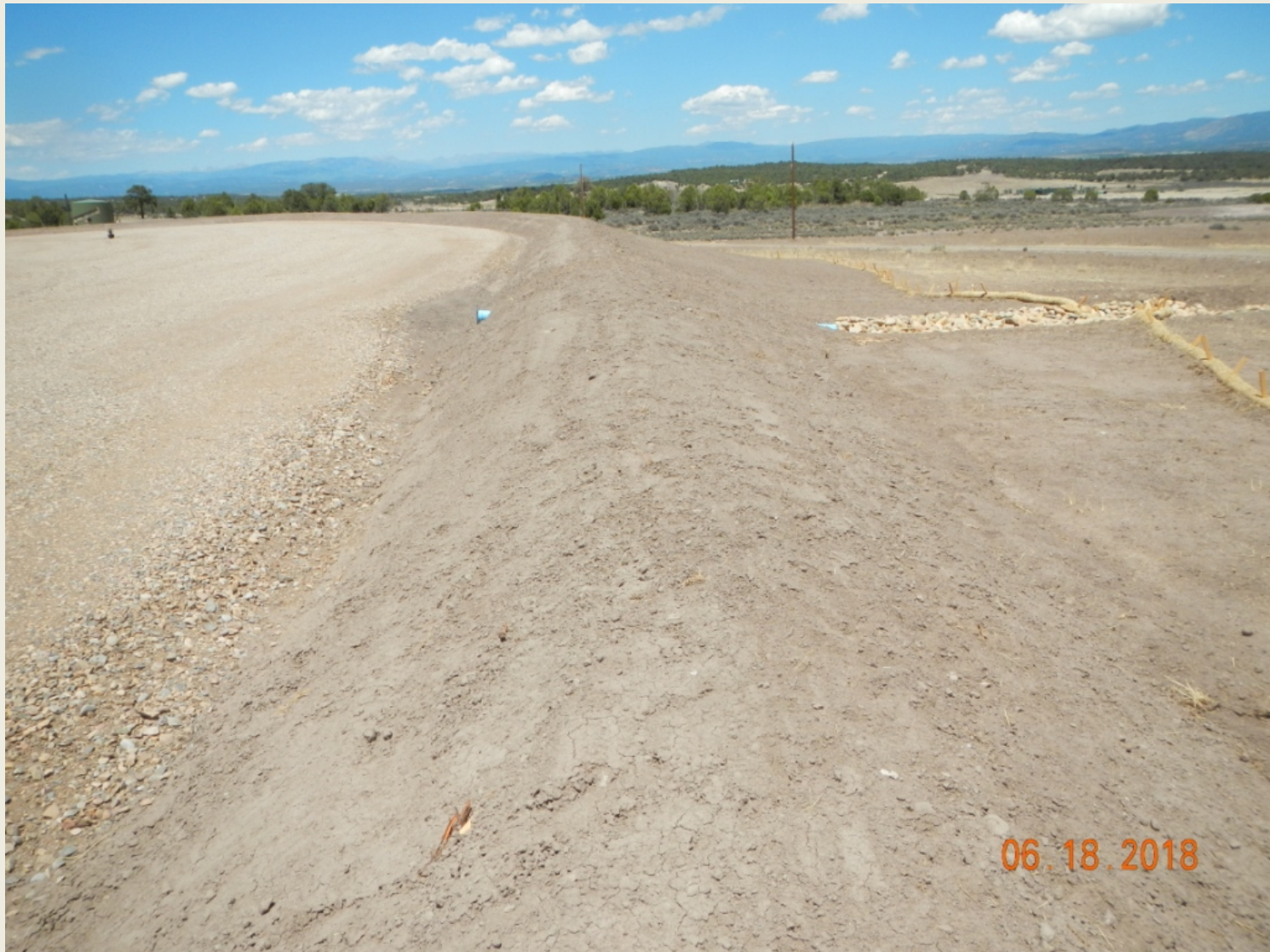
Photo 3. View of the portion of the project area from the southeastern corner facing northward. Berms and wattles in place. Erosion needs to be monitored until stabilization with vegetation is achieved.
