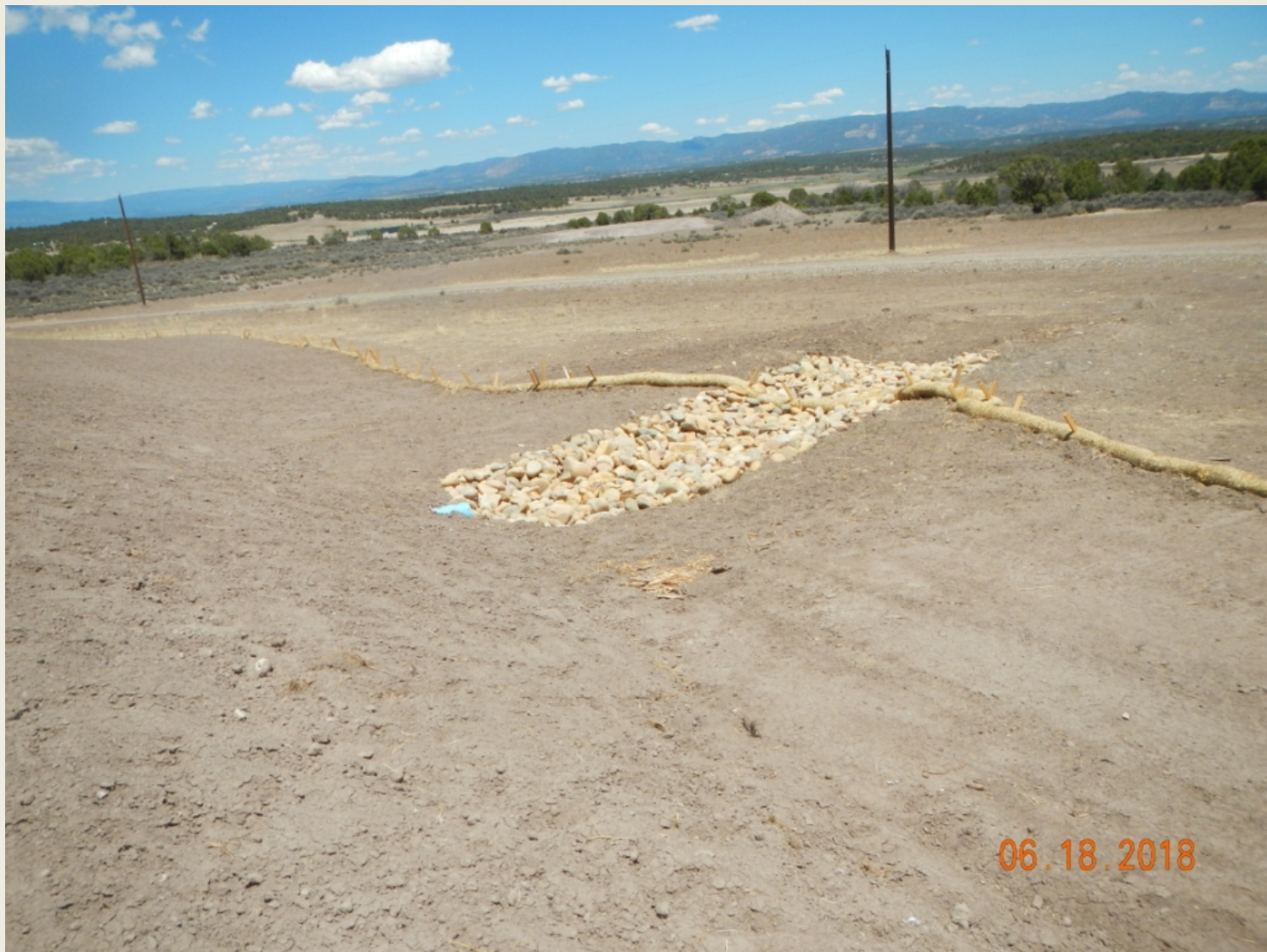
Photo 4. View of well pad drainage outlet armored with rock. Appears to be functioning.
