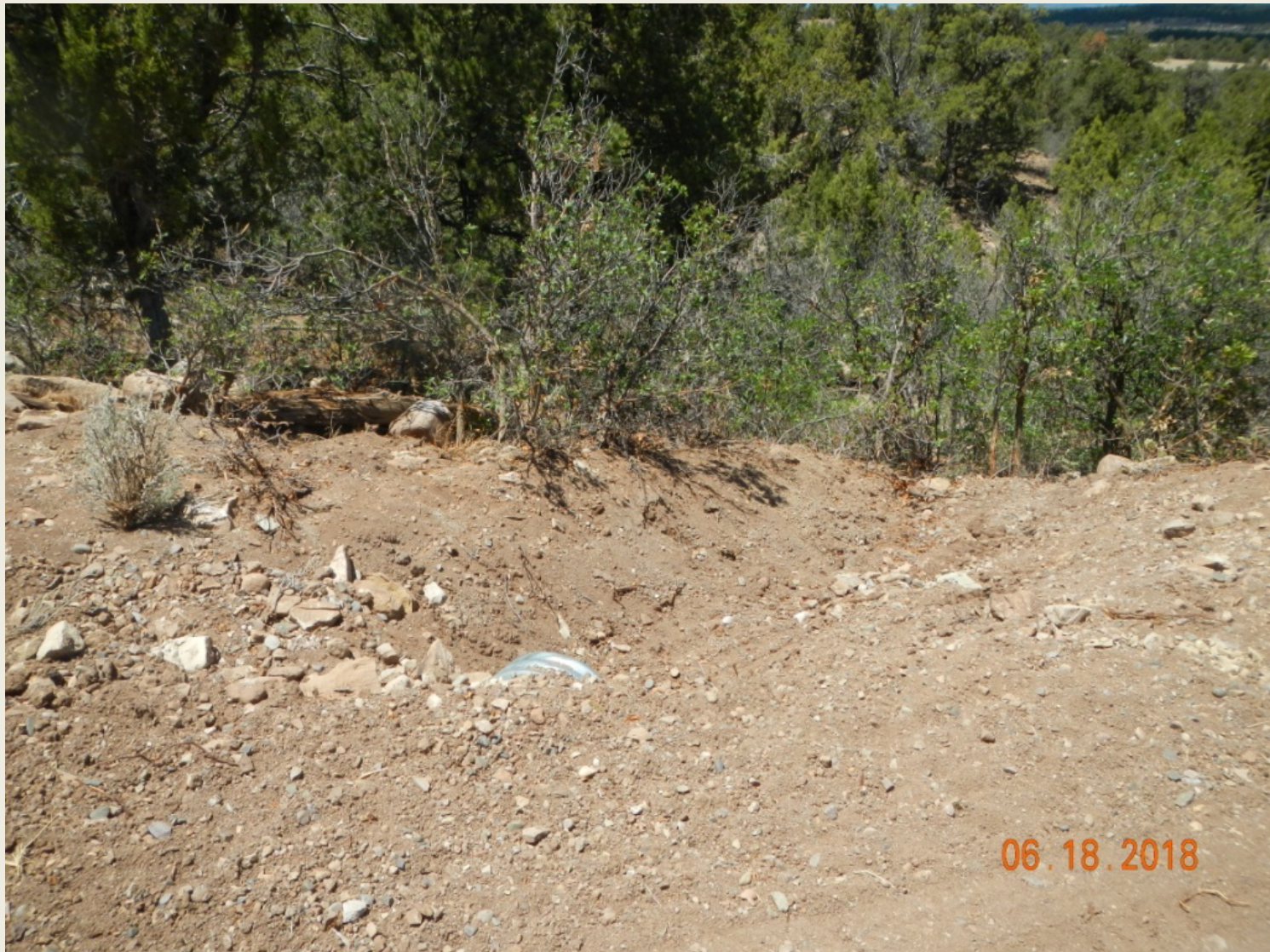
Photo 5. View of newly installed culvert outlet along the access road. It does not appear that stormwater flows exiting the culvert will be properly de-energized and will likely erode down the slope. Erosion and sediment controls should be installed to de-energize flows exiting the culvert and filter sediment. Loose soils need to be stabilized.
