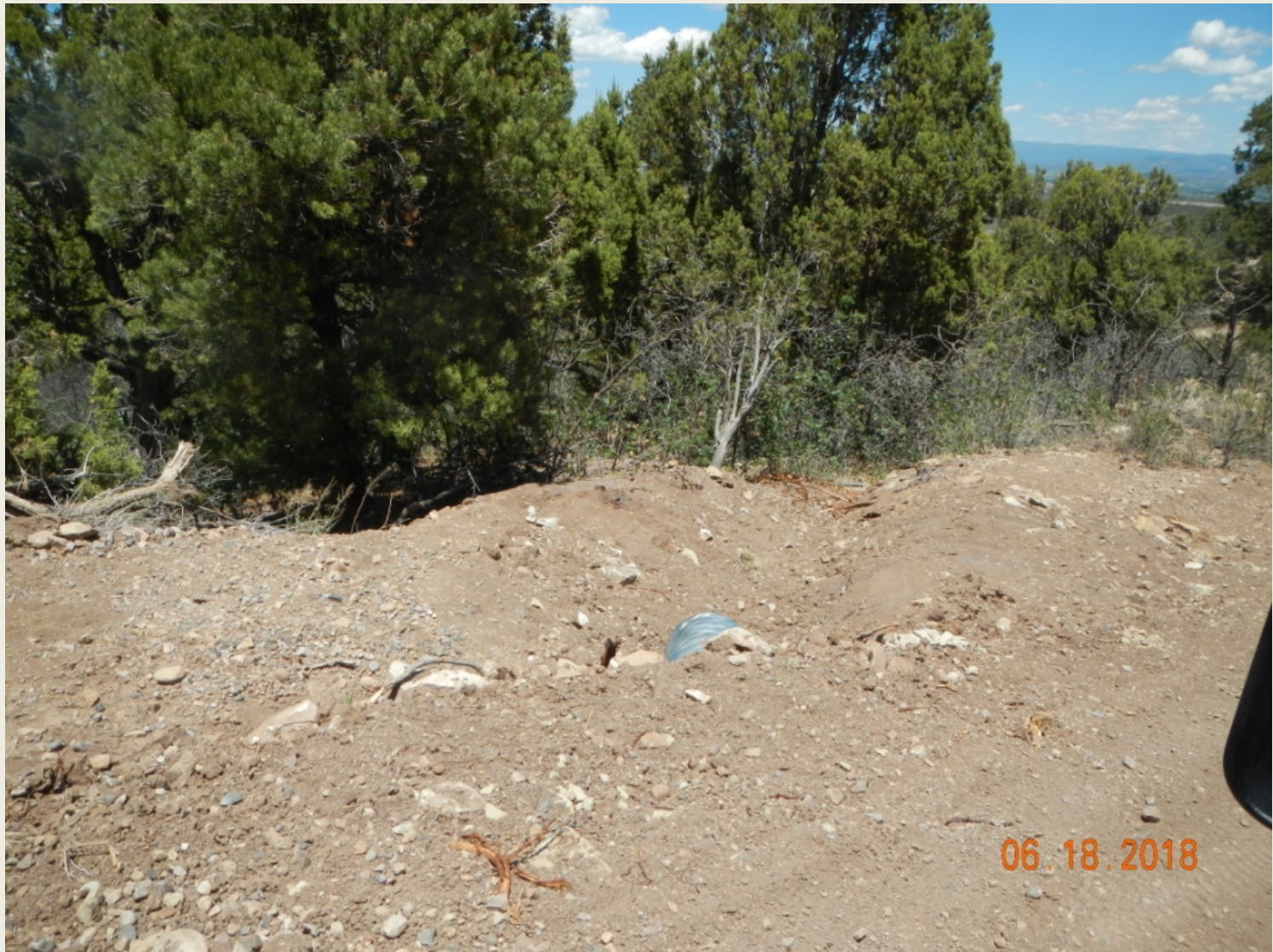
Photo 6. View of another newly installed culvert where loose soils are not properly stabilized and stormwater flows are diverted downslope without proper erosion and sediment controls.
