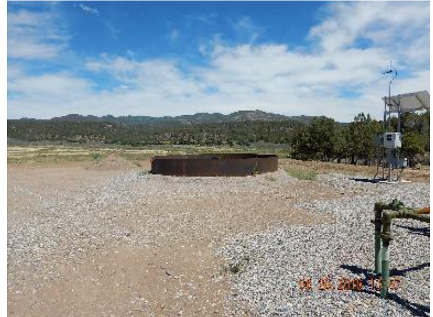
Photo 2: Production tank containment with no signage.
