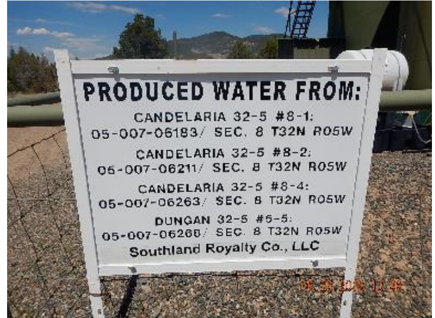
Photo 4: Tank battery sign.
