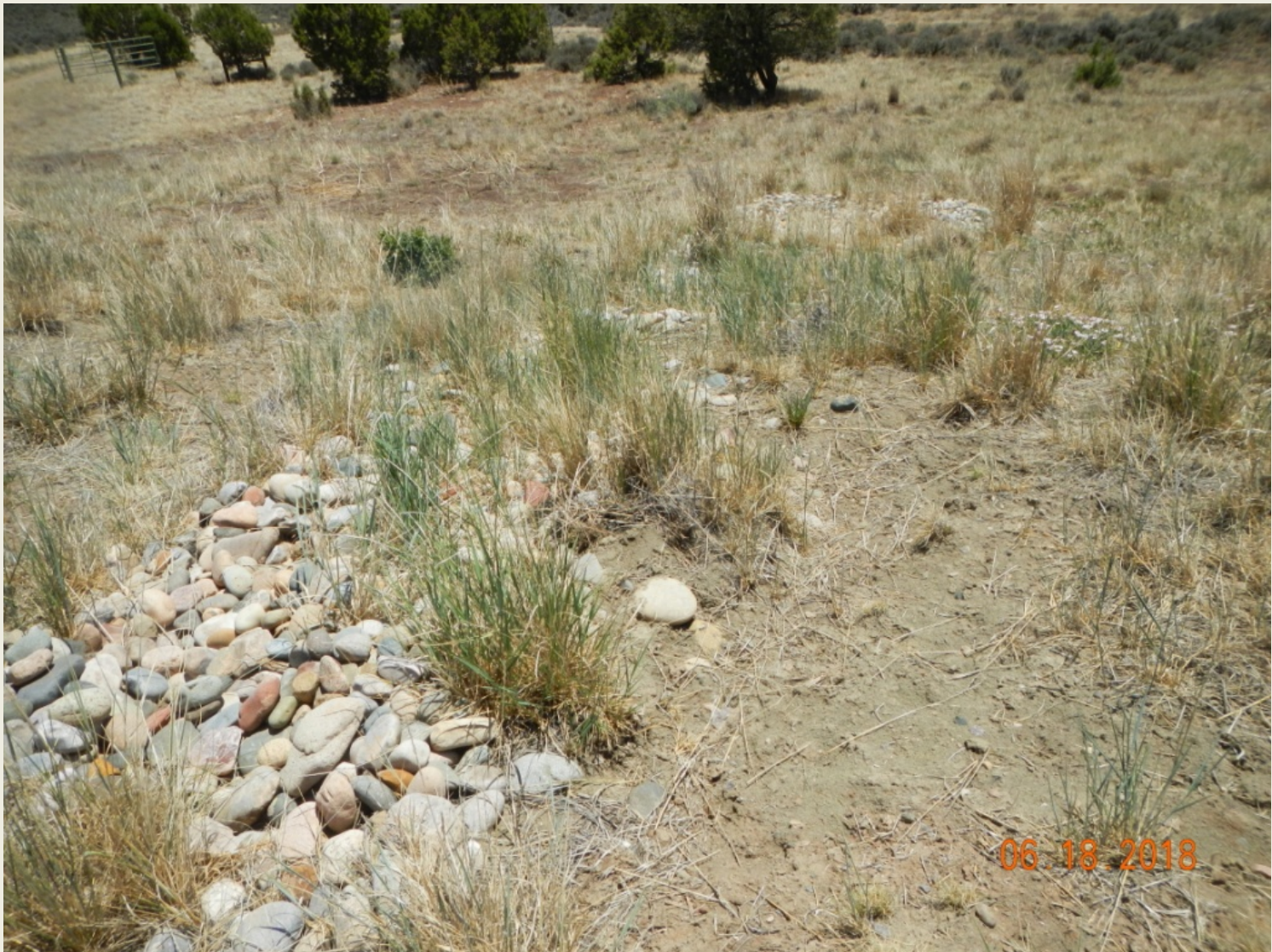
Photo 4. View of cobble run-down in the eastern portion of the project area. Appears to be functioning at this time.
