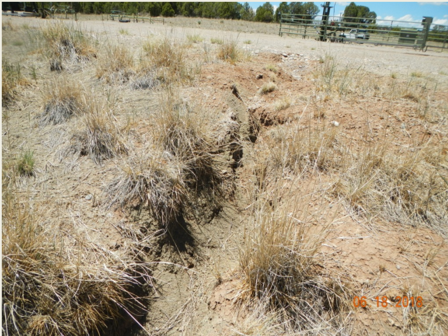
Photo 5. View of erosional channel approximately 2 feet wide and 2.5 feet deep in the eastern portion of the project area that needs stabilization.
