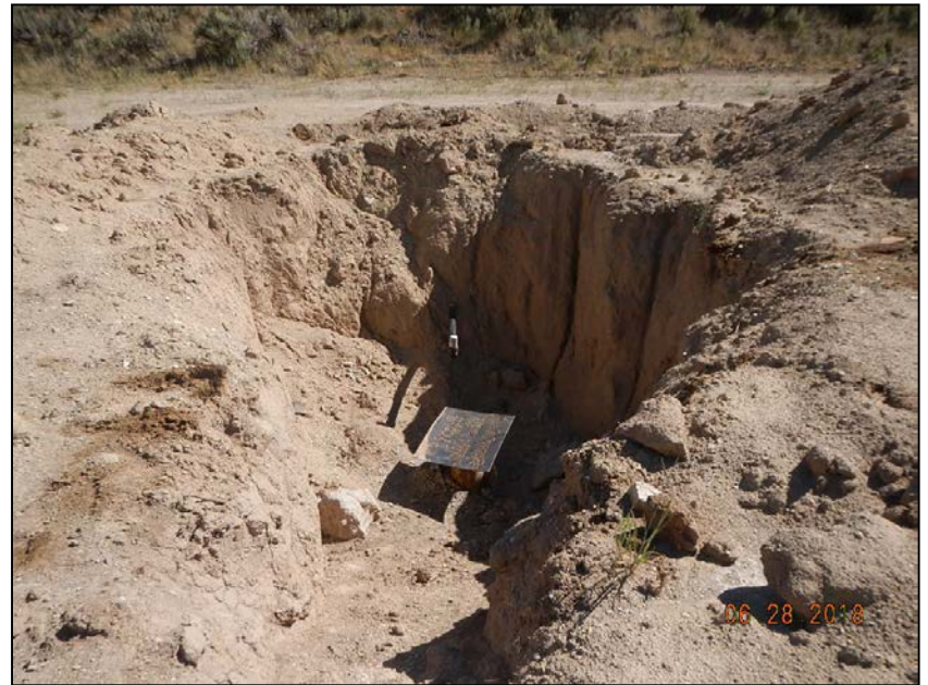
Photo 2. Excavation around cut off wellhead.
