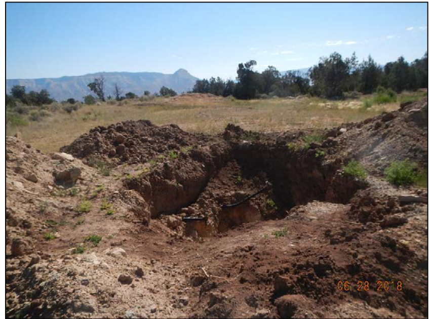
Photo 2. Excavation around cut off wellhead.
