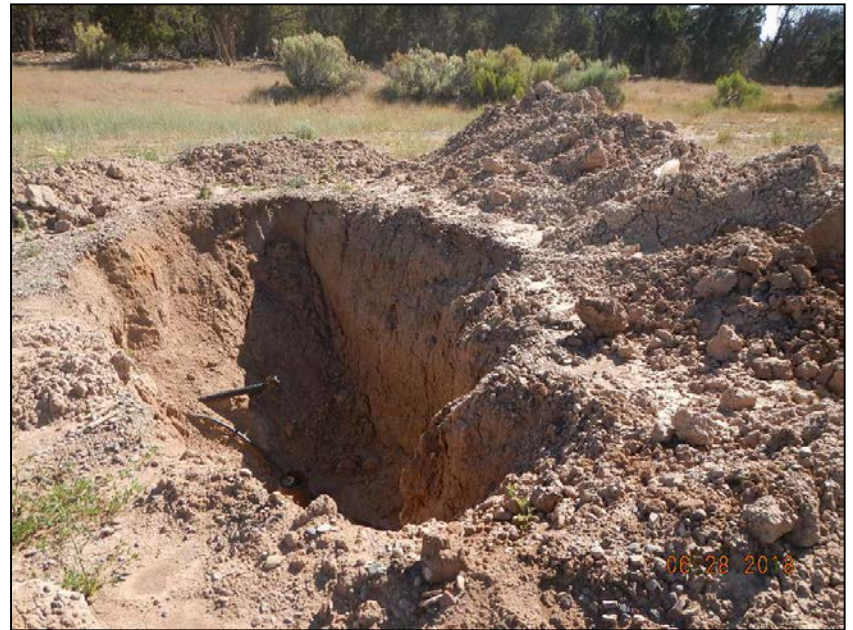
Photo 2. Excavation around cut off wellhead.
