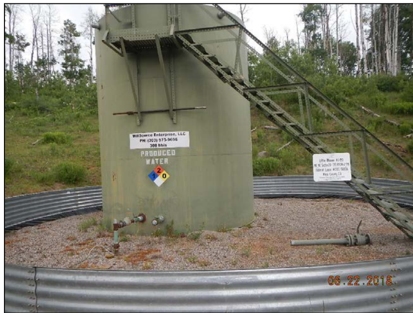
Photo 2. Tank and signs.
