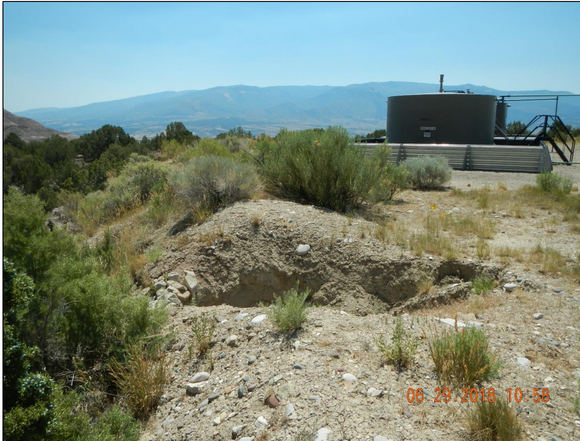
Washing check dam in north east corner of location.
