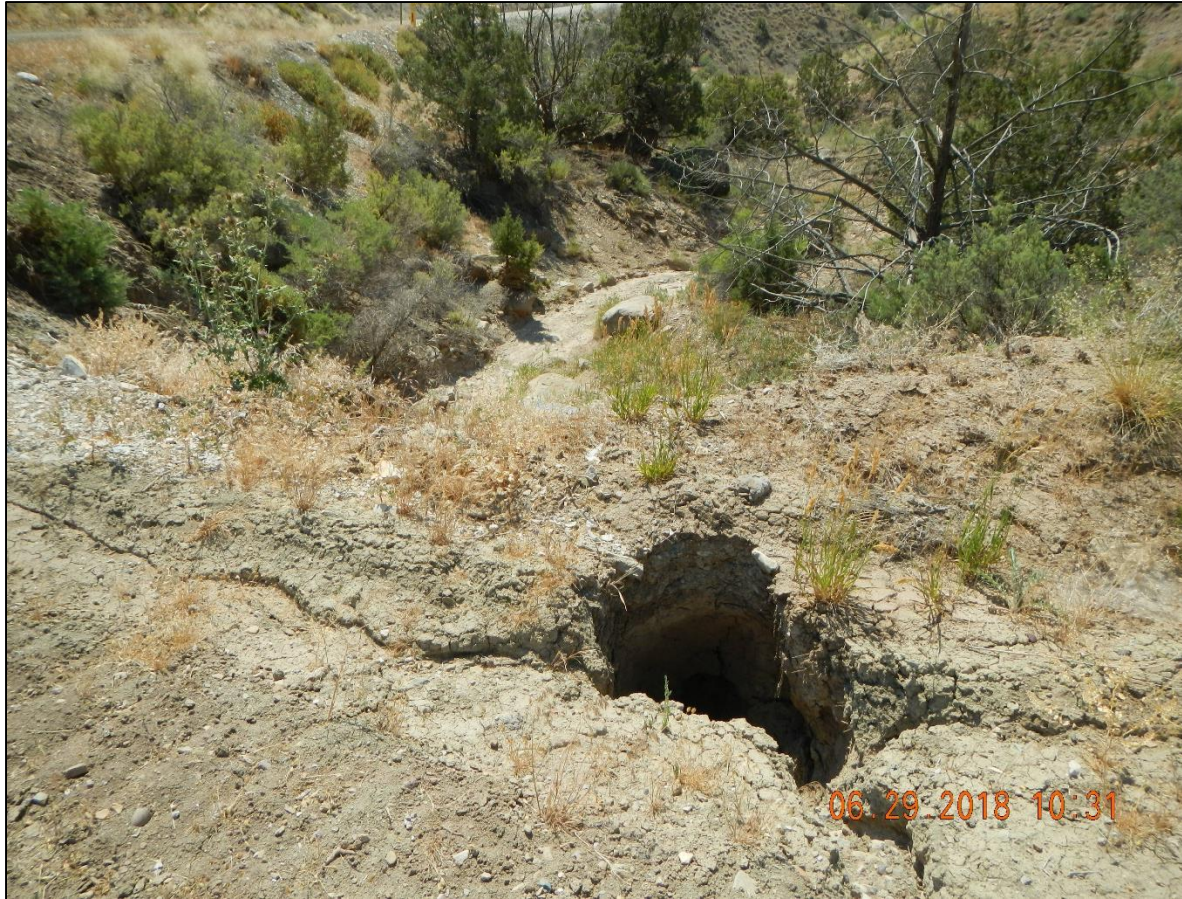
Washed hole at switch back (39.47929 -108.06580)
