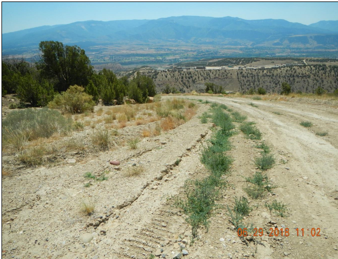
Washing ruts and rills on access road.
