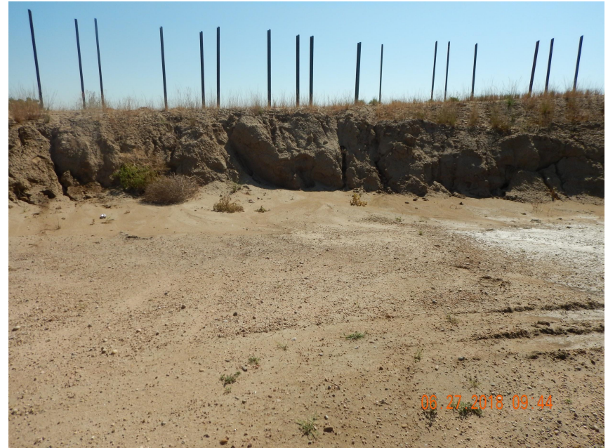
Photo 17. Photo taken from the northeastern well pad, facing East. Photo illustrates rill and gully erosion on the eastern earthen berm. See comments under Photo 16.
