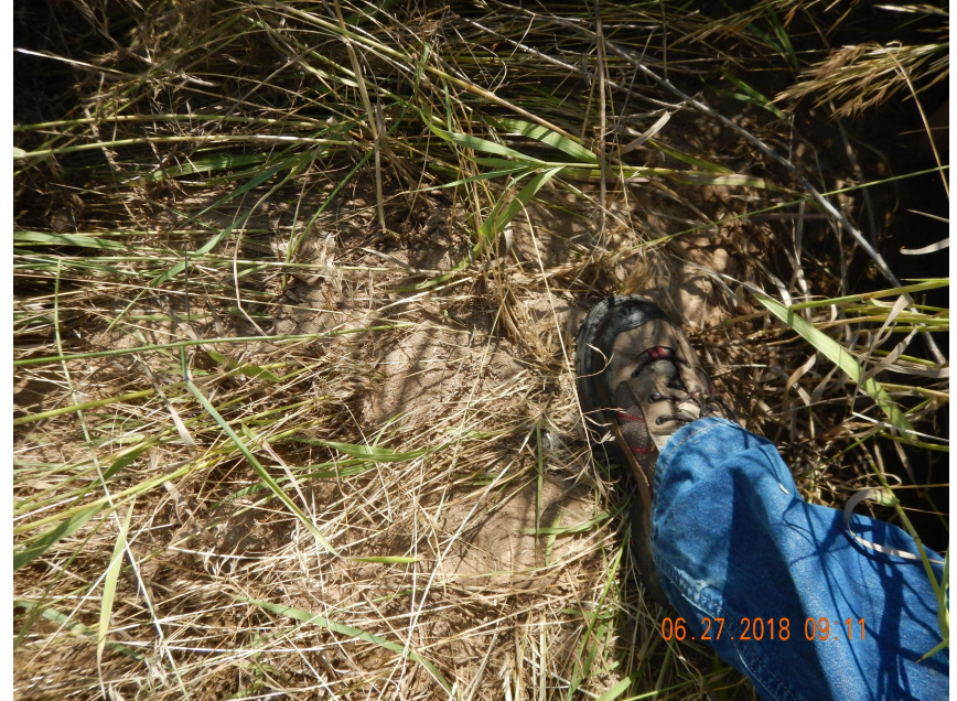
Photo 4. Photo illustrating sediment discharge beyond the S-fence.
