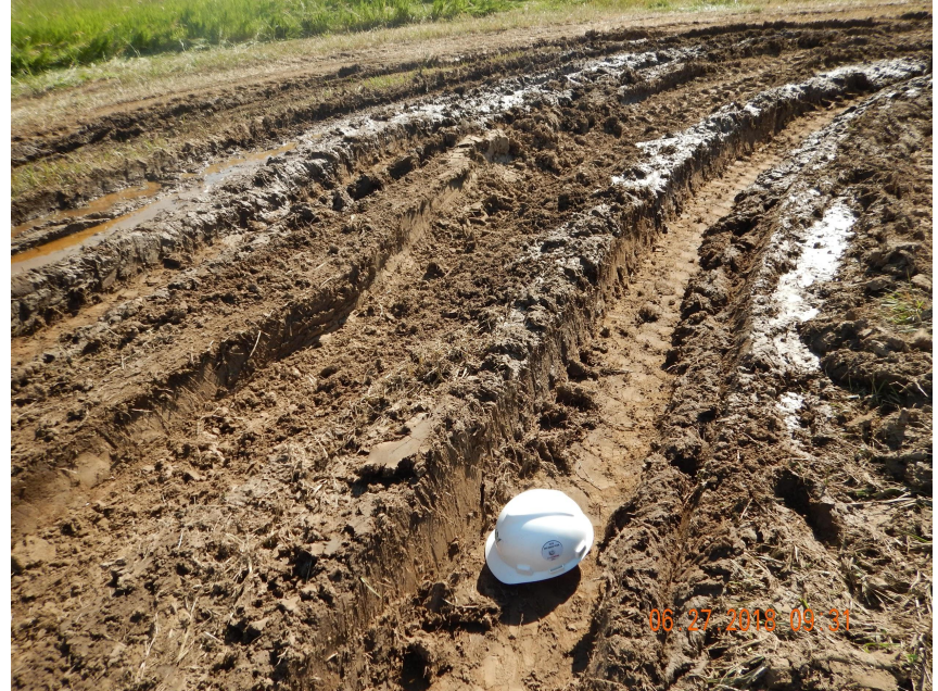
Photo 15. Photo taken from the northeastern perimeter of location, facing East. Photo illustrates rutting from equipment traffic due to sound wall removal.
