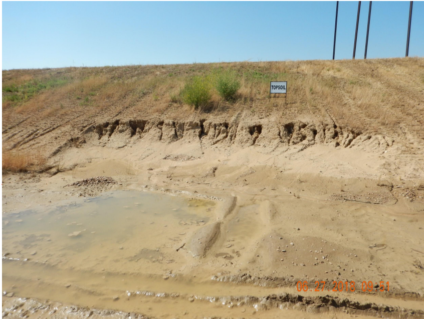
Photo 20. Photo taken from the southern well pad, facing South. Operator has failed to protect the topsoil stockpile from erosion per Rule 1002.c.
