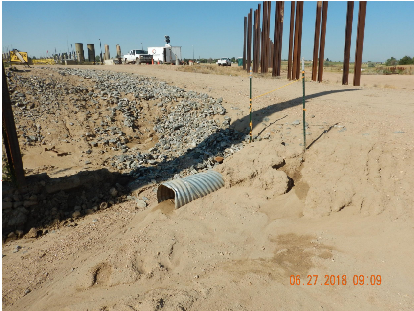
Photo 5. Photo taken from the east side of the entrance to the facility location, facing West. Rill erosion and sediment accumulation observed. Stormwater BMP maintenance in need of repair.
