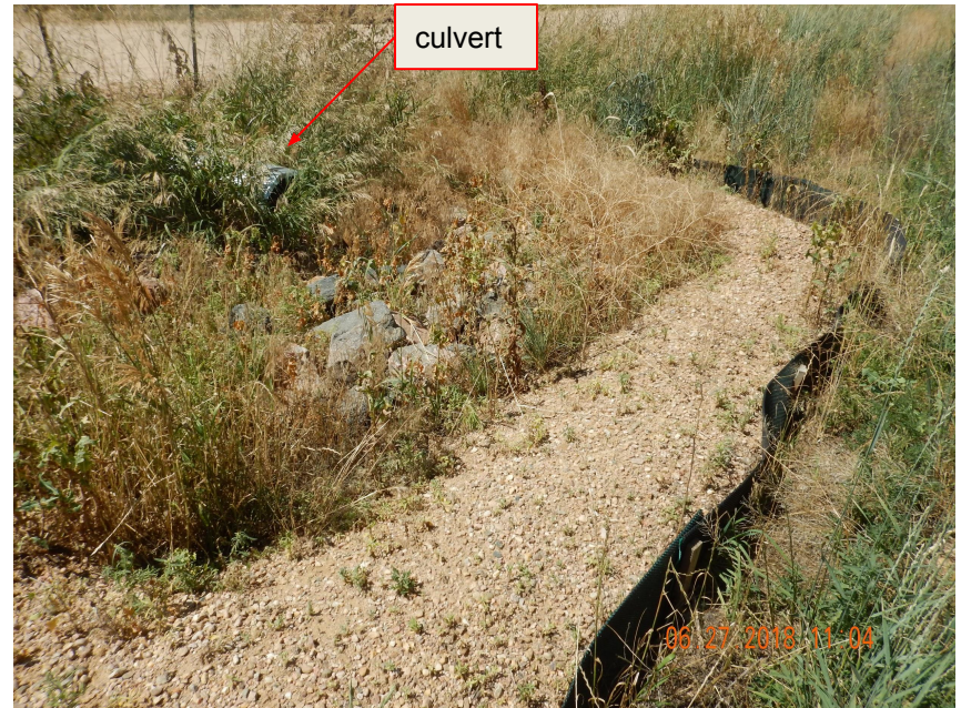
Photo 2. Photo taken along a portion of the access road. Photo illustrates a stabilized outlet area installed in conjunction with a culvert. No sediment discharge was observed beyond the stabilized outlet area. Note: Straw wattles along the access road are in need of maintenance.
