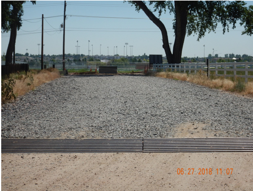
Photo 1. Photo taken from the entrance of location off 71st Ave., facing East. Vehicle tracking device installed and appears to be in proper functioning condition.
