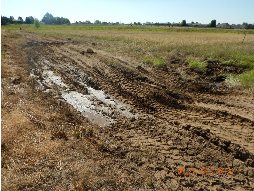
Photo 12. Photo taken from the southern perimeter of location, facing East. Surface damages due to sound wall removal shall be repaired and reclaimed. Note: Surface disturbance due to sound wall removal was observed outside of the permitted area along the west, east and northeastern areas.
