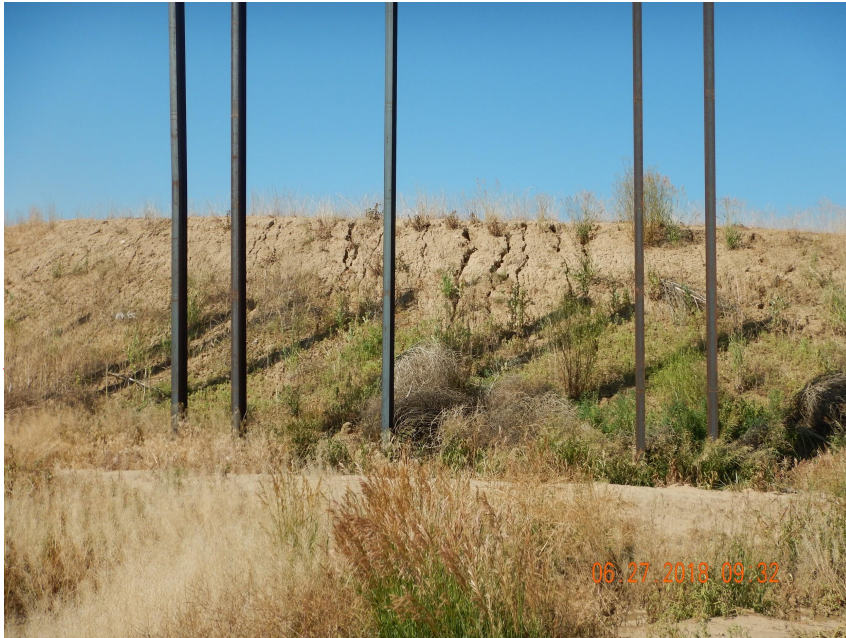
Photo 16. Photo taken from the northeastern perimeter of location, facing South. Photo illustrates rill erosion on the eastern earthen berm that has not been maintained to reasonably minimize erosion and site degradation per Rule 1002.e.
