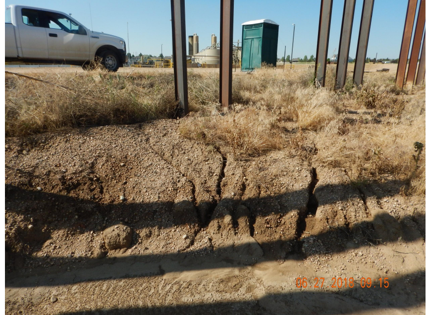
Photo 8. Photo taken from the northwestern perimeter of location, facing South. Rill erosion was observed along the northern perimeter of the location. Ditch BMP in need of maintenance from rill erosion off the northern perimeter. Note: Weed debris (Kochia weeds) was observed along portions of the perimeter and shall be controlled and managed per Rule 603.f.
