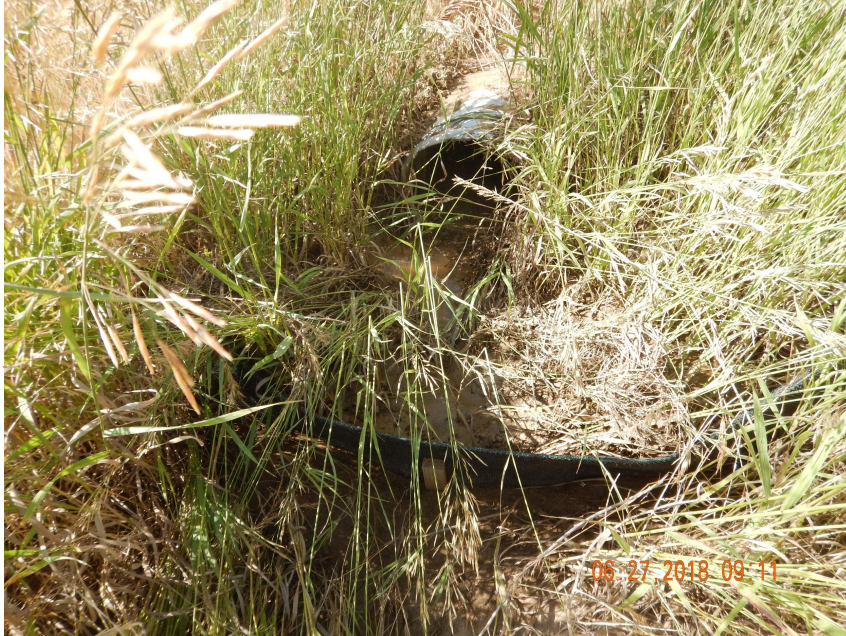
Photo 3. Photo taken from the northwestern discharge point. S-fence was installed to outlet protection in conjunction with the culvert. Sediment discharge was observed beyond the S-fence.
