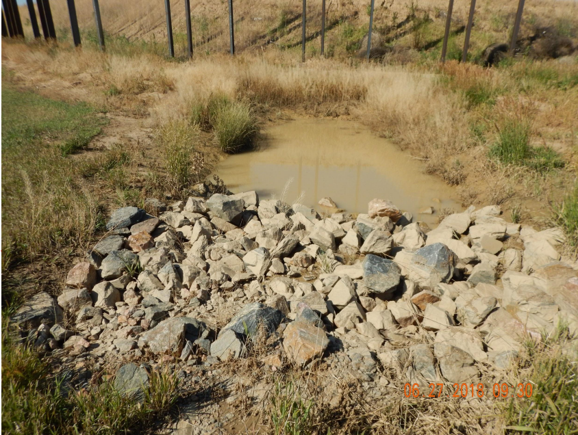
Photo 14. Photo taken from the northeastern perimeter of location, facing Southwest. Appears some sediment discharge was observed beyond the stabilized outlet area.
