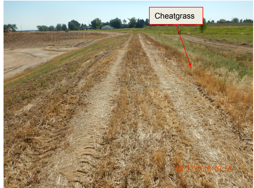
Photo 21. Photo taken from the topsoil stockpile, facing East. Operator has failed to protect the topsoil stockpile from compaction and weed establishment. Appears the Operator only seeded the north-facing slope while the south-facing slope has cheatgrass establishment.
