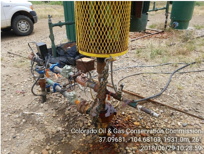
Photo 1. Wellhead/packing leak
