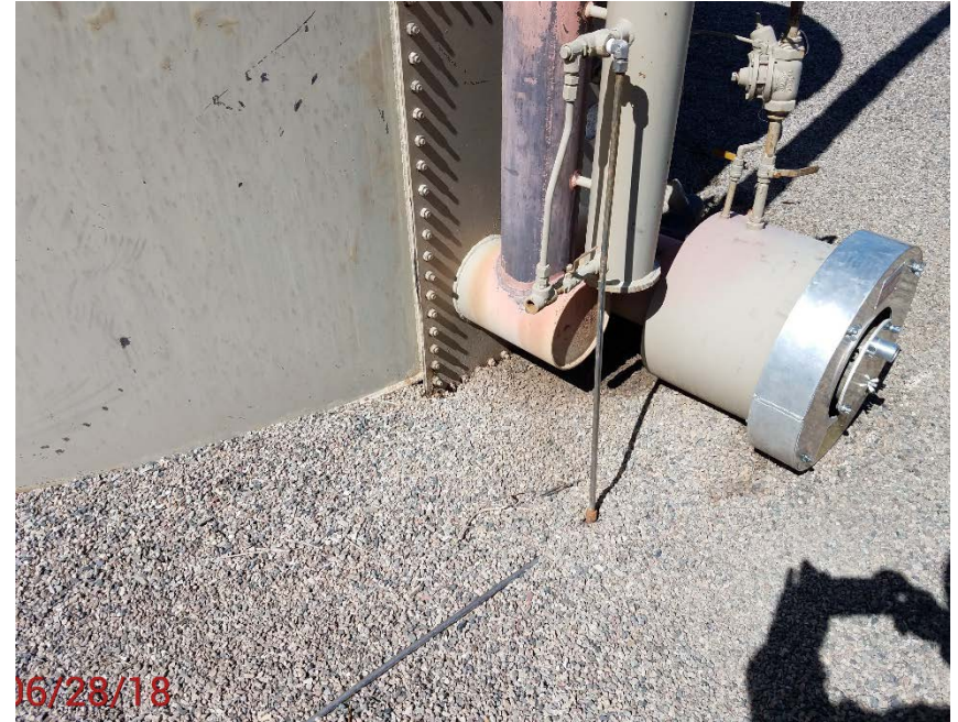
Location Photo #8, Stained rock in containment under tank heater.
