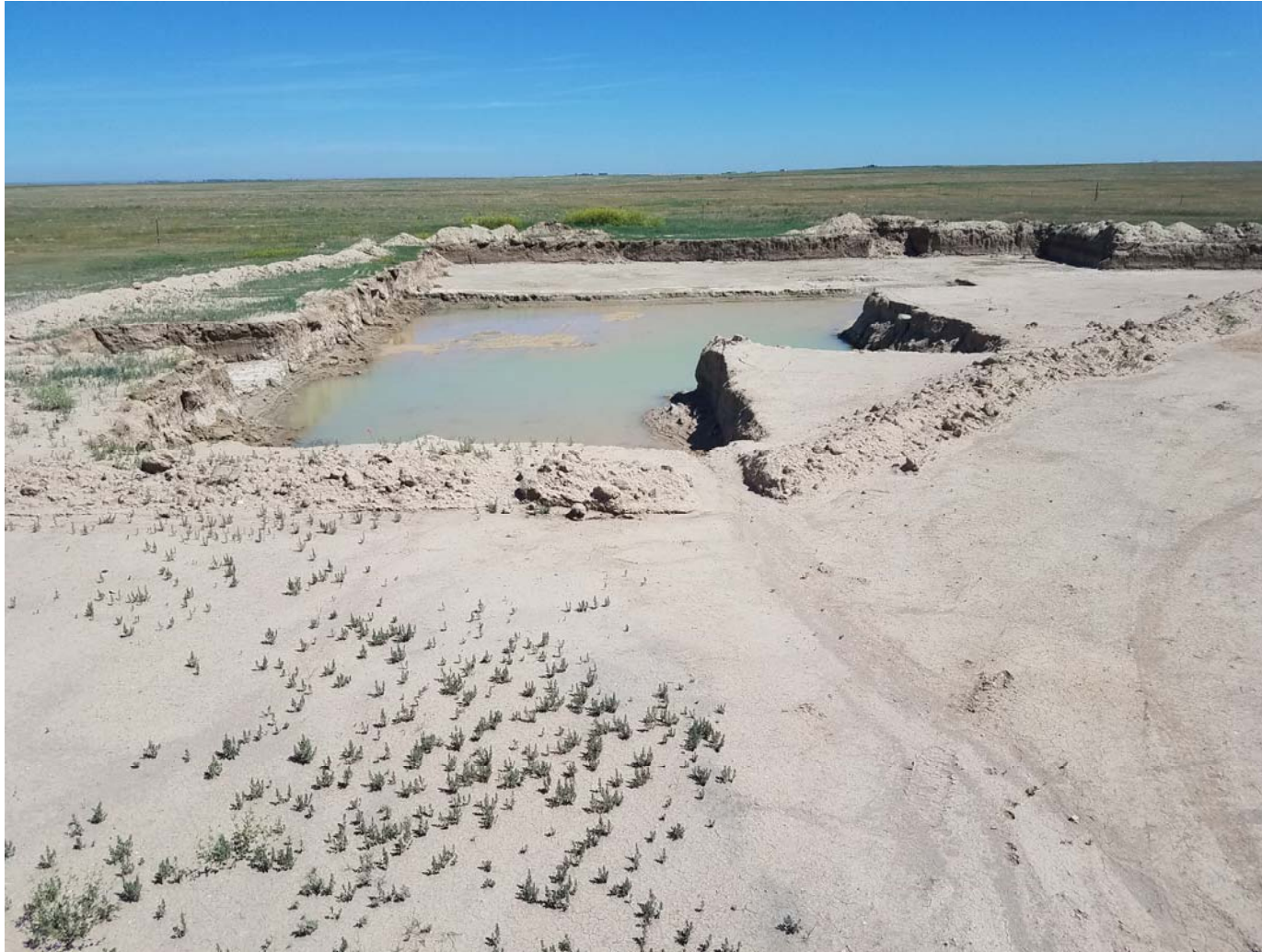
Photo 1 – Croissant #1 wellhead release, spill ID 454027, backfilled in process. Looking north.
