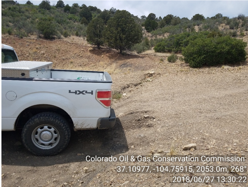
Storm water damage at location entrance
