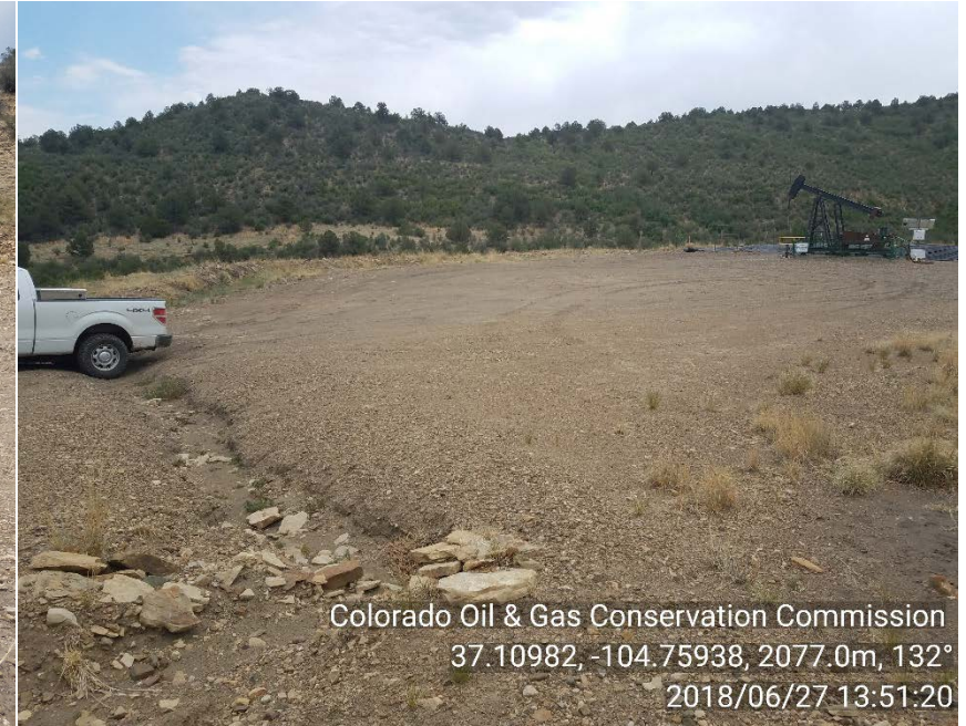
Storm water damage at entrance of location
