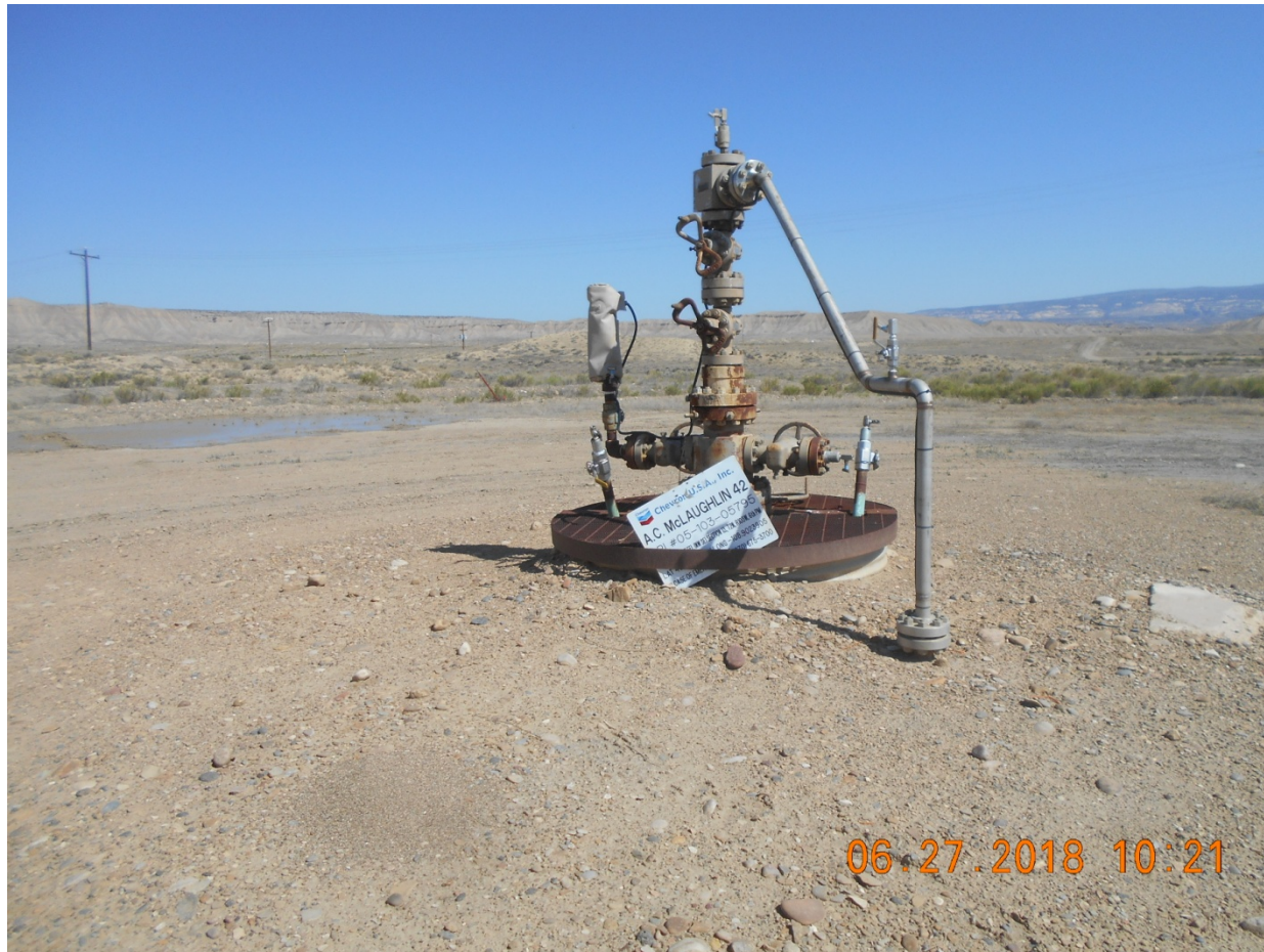
Injection wellhead.
