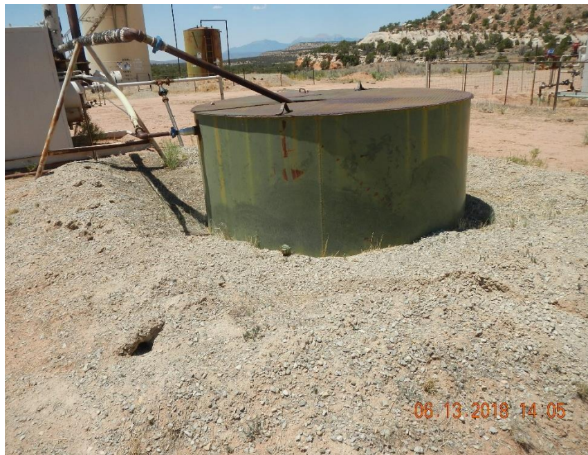
Damaged earthen berm for open topped tank. Tank does not have label or placard.
