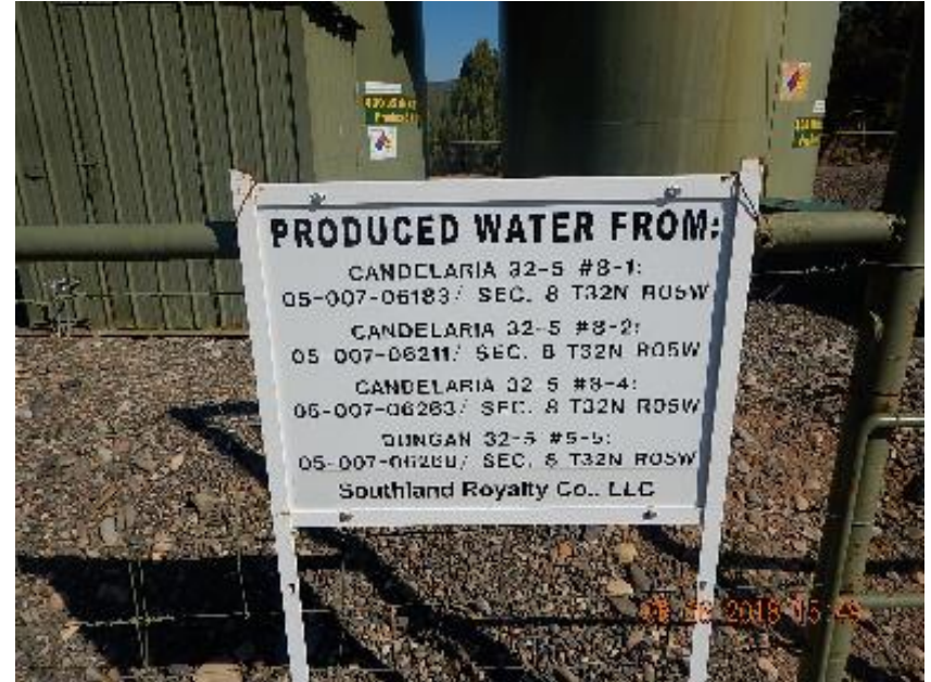
Photo 8: Tank battery sign..
