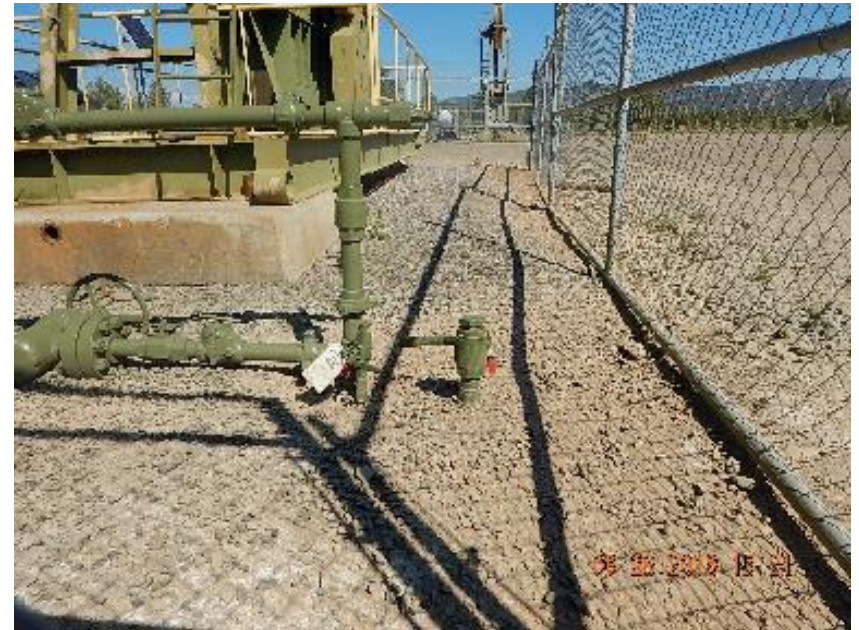
Photo 2: Unused 1" (A) point and unused 2" (A) point steel risers at #5-5 wellhead.
