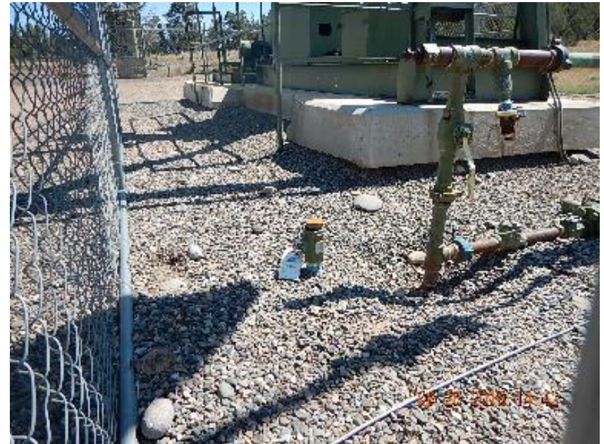
Photo 2: Unused 2" steel riser (A) point at wellhead.
