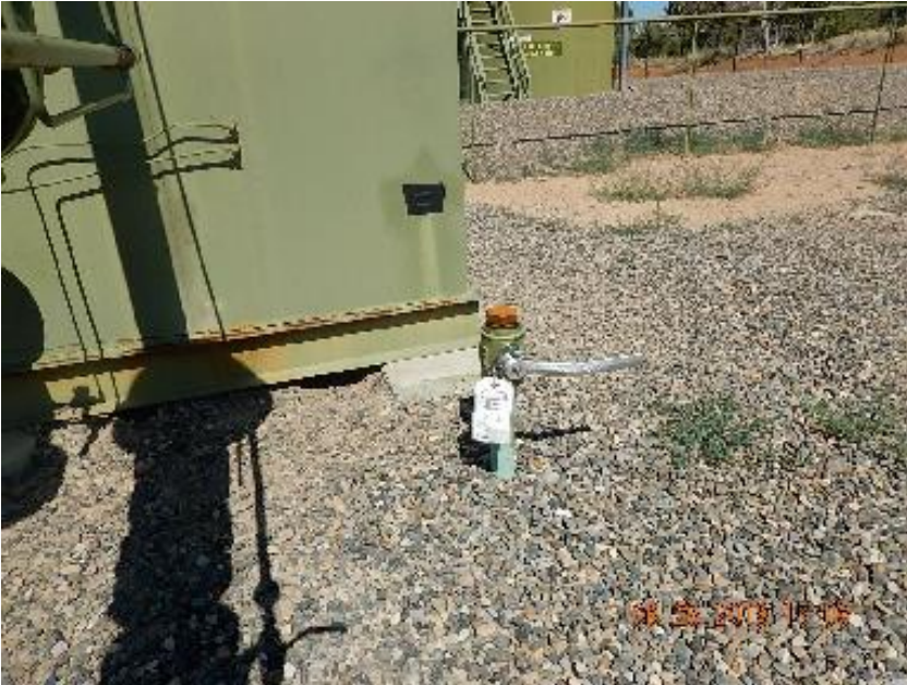
Photo 3: Unused 2" steel riser (B) point at separator.
