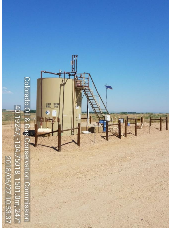
Photo 1 Tank Battery
