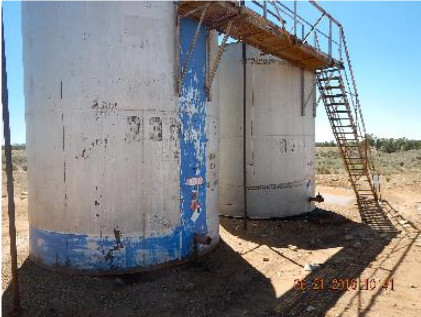
Photo 3: Tank battery overview.
