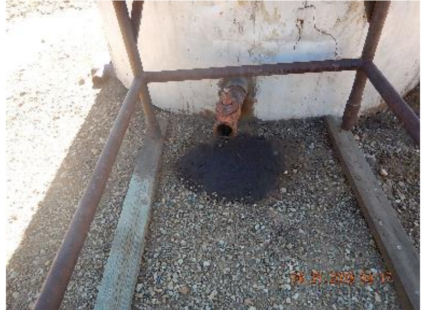
Photo 4: Impacted soil at tank load out..
