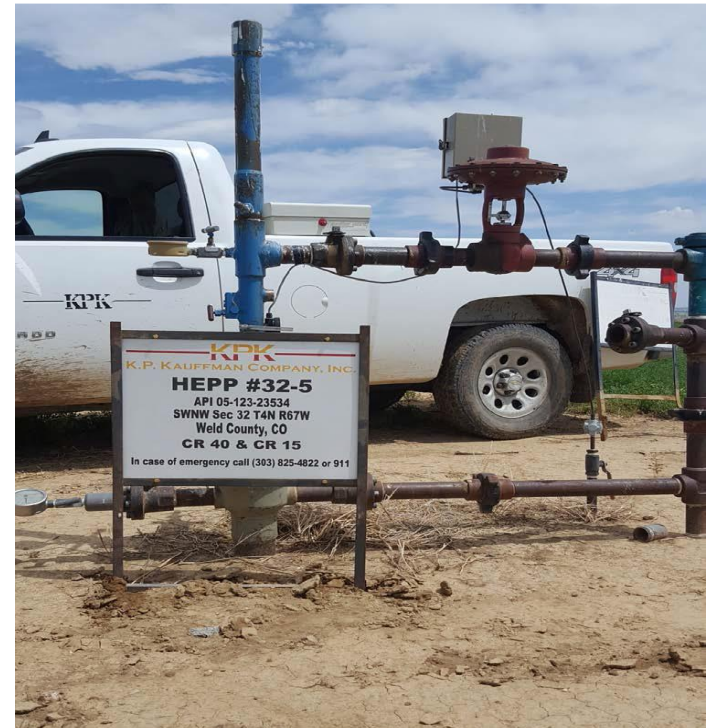
Sign after completed CA
