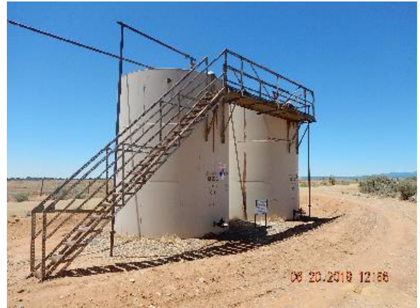
Photo 2: Tank battery overview.
