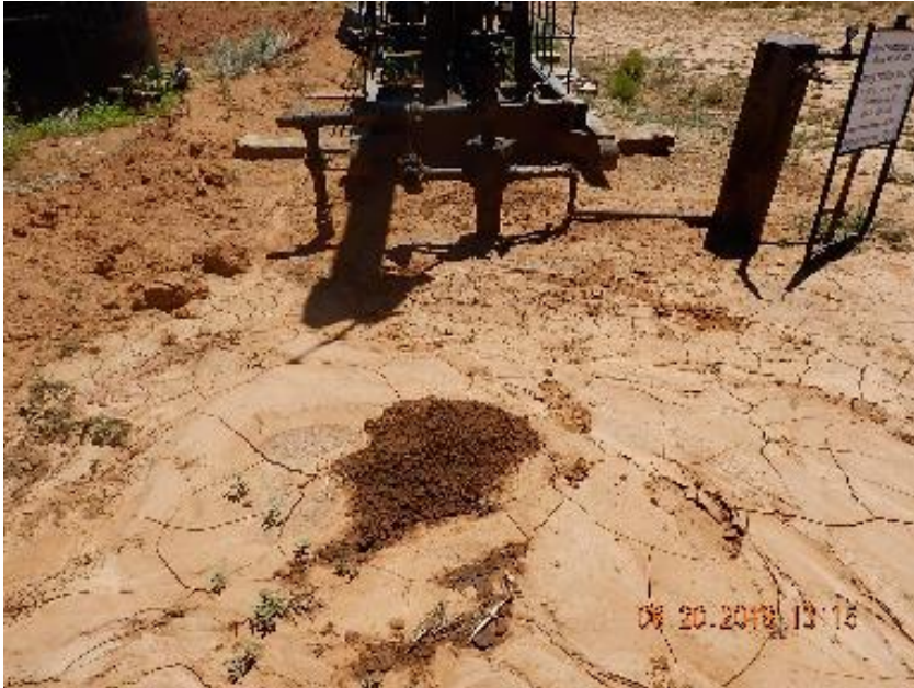
Photo 3: Impacted soil at wellhead.
