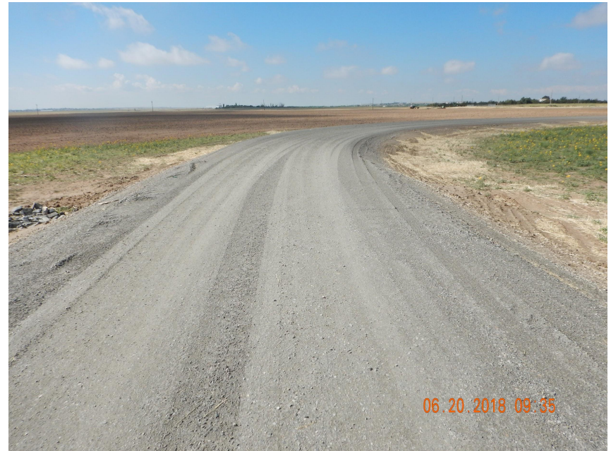
Photo 2. Photo taken from the entrance of location, facing South. Photo illustrates a portion of the access road which has been gravelled.
