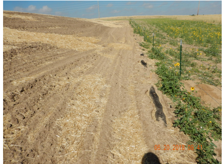
Photo 6. Photo taken from the northern perimeter of the location, facing West. Appears soil material was pushed over the top of the wattle BMP from equipment traffic which is no long in proper functioning condition.
