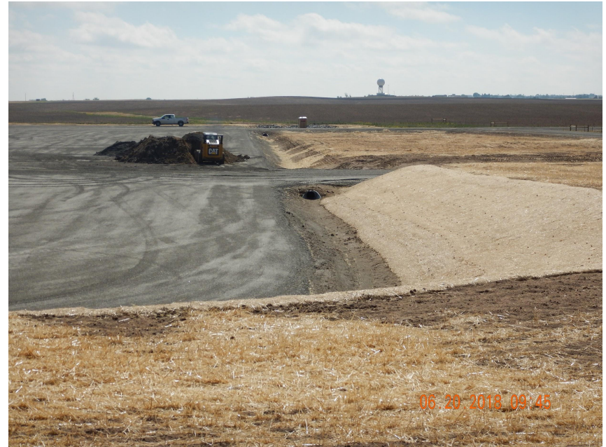
Photo 10. Photo taken from the southwestern perimeter of the location, facing East. Photo illustrates well pad operational areas have been stabilized with gravel, as well as cut slopes with erosion control blankets.
