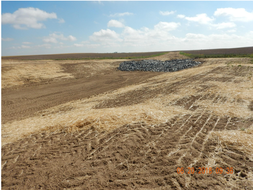
Photo 3. Photo taken from the southeastern perimeter of the location, facing East. Photo illustrates the sediment trap BMP. A ditch BMP has been installed along portion of the perimeter of the location which is directed to this sediment trap. Disturbance areas have been mulched and crimped, and appear to be seeded. Crimped mulch does not appear to be crimped along portions.
