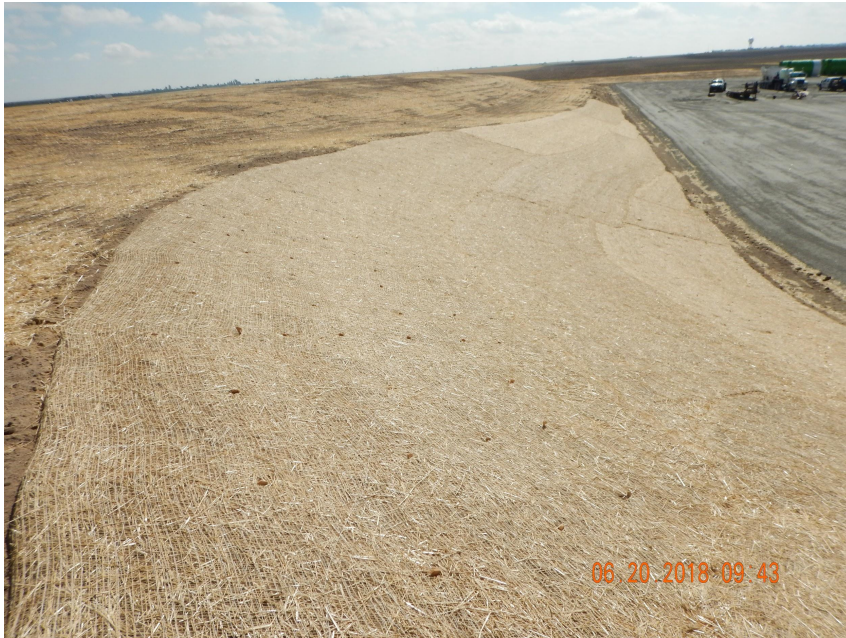
Photo 7. Photo taken from the northwestern perimeter of the location, facing East. Cut slope has been stabilized with erosion control blankets.
