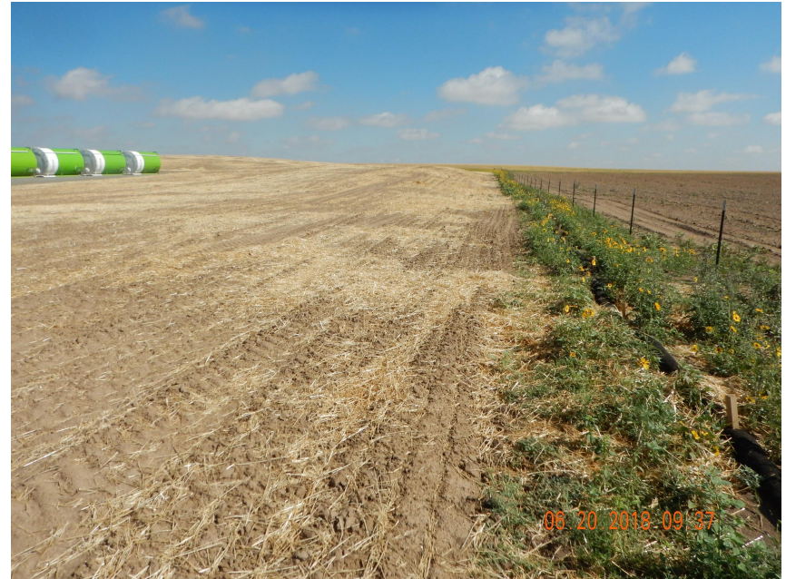
Photo 4. Photo taken from the southeastern perimeter of the location, facing North. Filtrexx wattle has been installed along portions of the perimeter of the location. Topsoil appears to be stored along the eastern perimeter of the location.
