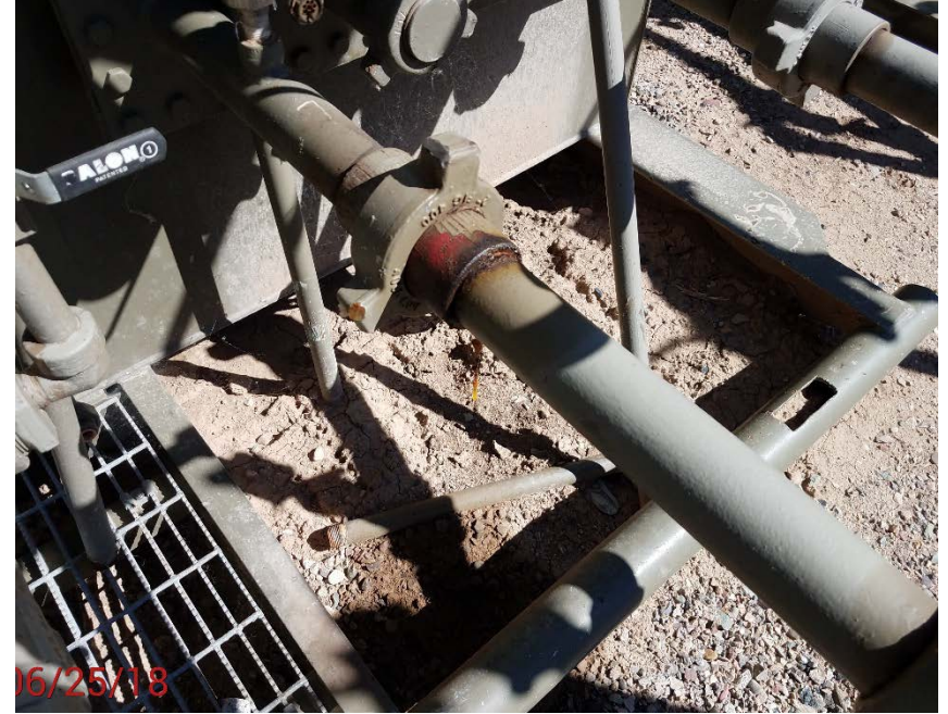
Location Photo #7, Small drip on a flowline
