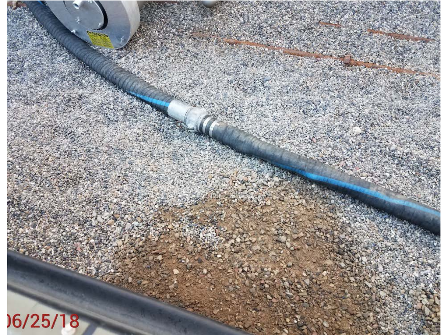
Location Photo #5, Stained material in battery containment
