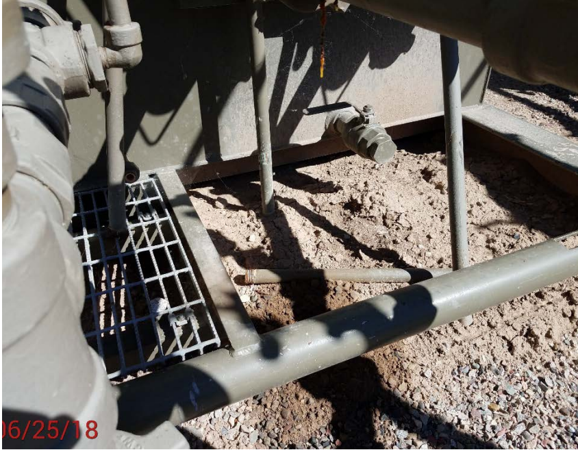
Location Photo #6, Small drip on a flowline from a separator
