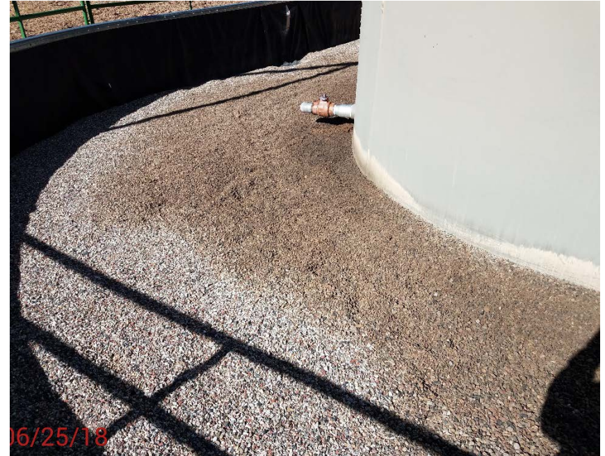
Location Photo #2, Stained rock in battery containment
