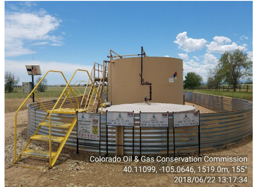
Photo 2. Tank battery
