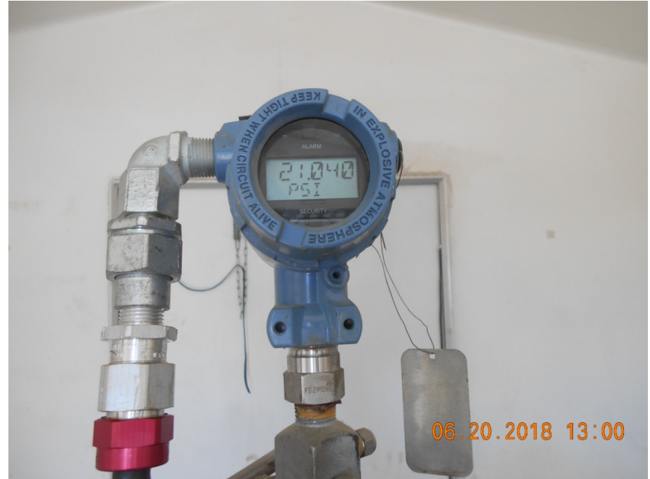
Injection wellhead tubing gauge
