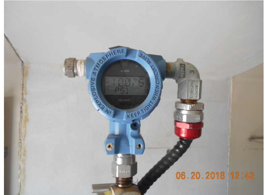
Injection wellhead tubing gauge
