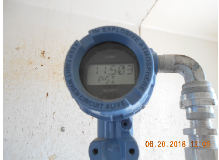
Injection wellhead tubing gauge
