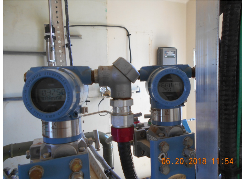
Injection wellhead tubing gauge
