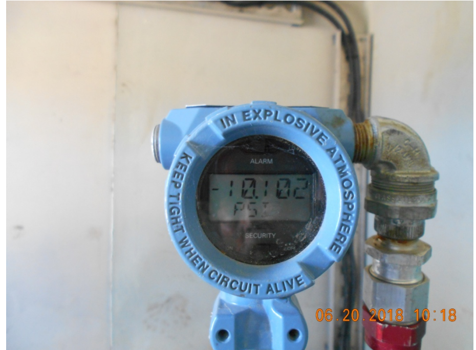
Injection wellhead tubing gauge
