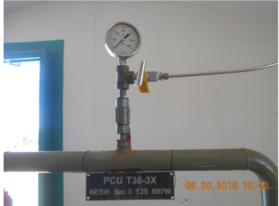
Injection wellhead tubing gauge
