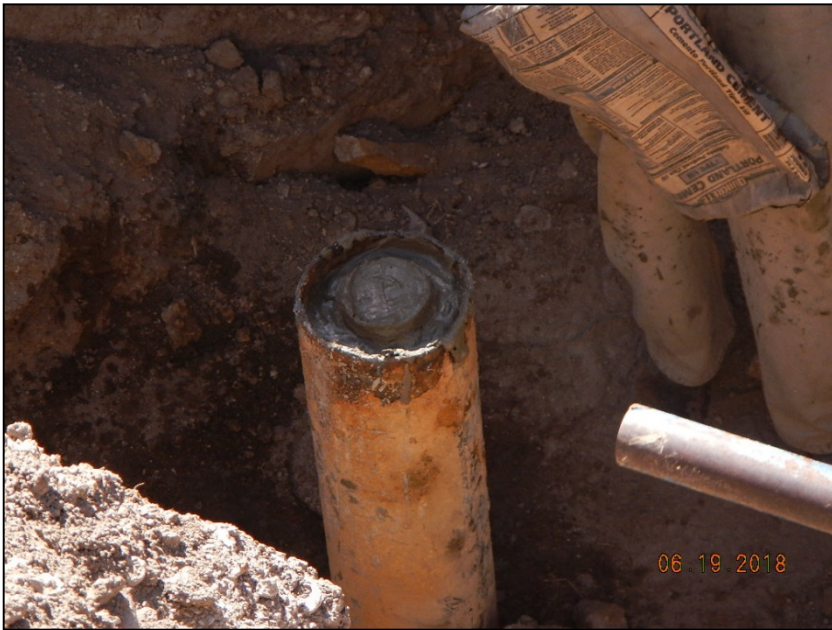
Photo 1. Cement to surface.
