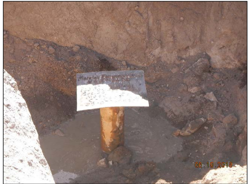
Photo 2. Plate welded on.
