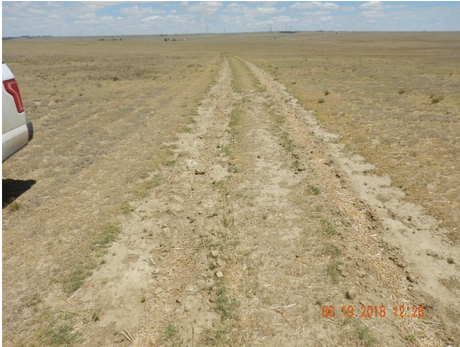
Photo 1: Photo taken from the access road, facing northeast. Photo shows no additional work appears to have been conducted since the previous inspection; it appears a two-pronged ripper only cut through areas of the ruts within the road. Compaction alleviation does not appear to have been conducted in accordance to reclamation requirements. Compaction concerns remain on access road.
