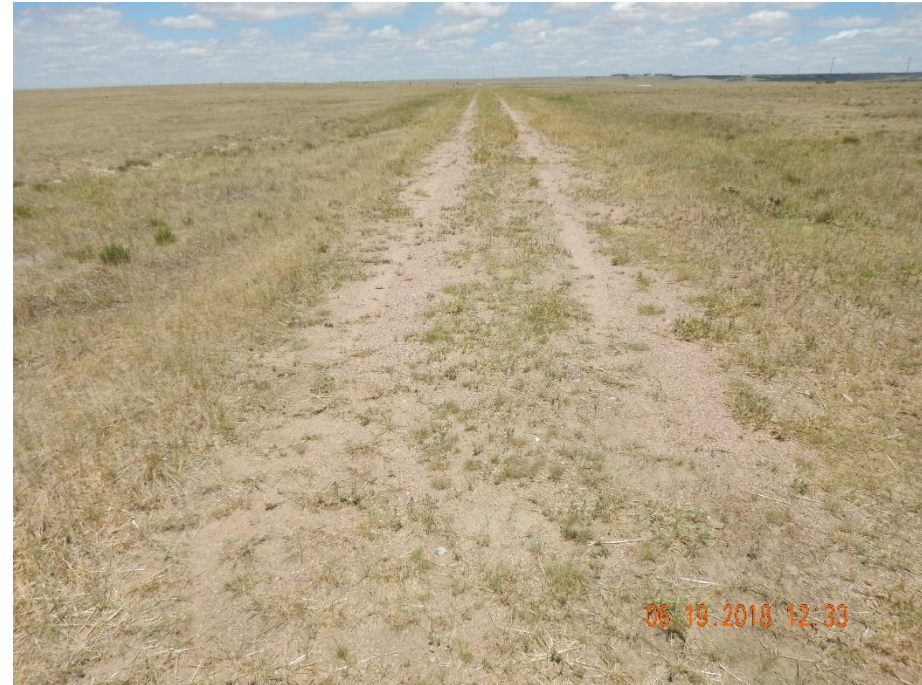
Photo 4: Photo taken from the northern portion of the access road. Photo shows portion of access road where no reclamation activities appear to have been conducted; gravel remains on road, access road has not been re-contoured, re-graded or had compaction alleviation conducted.
