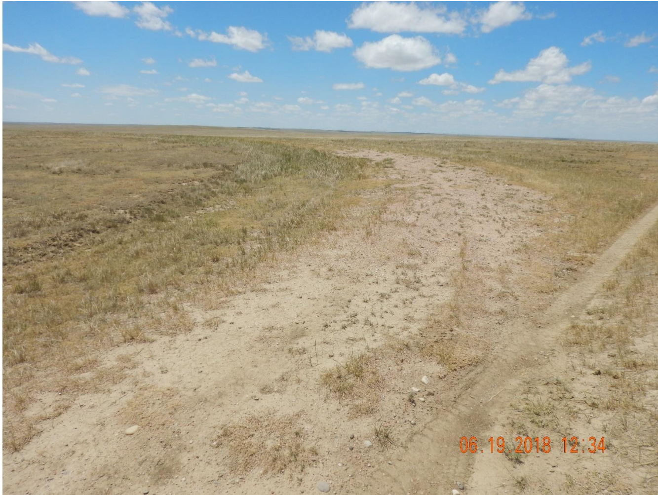
Photo 5: Photo taken from the area where the north section of access road joins the east/west ranch road, facing southwest. Photo shows portion of access road where no reclamation activities appear to have been conducted; gravel remains on road, access road has not been re-contoured, re-graded or had compaction alleviation conducted.
