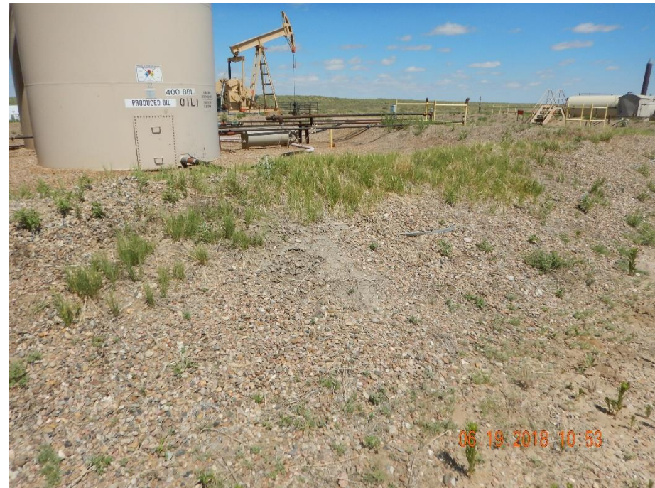
Photo 4: Photo taken from the east end of the tank battery berm, facing northwest. Photo shows vegetation establishment on the berm. Vegetation compromises the integrity of the containment berms and needs to be removed.
