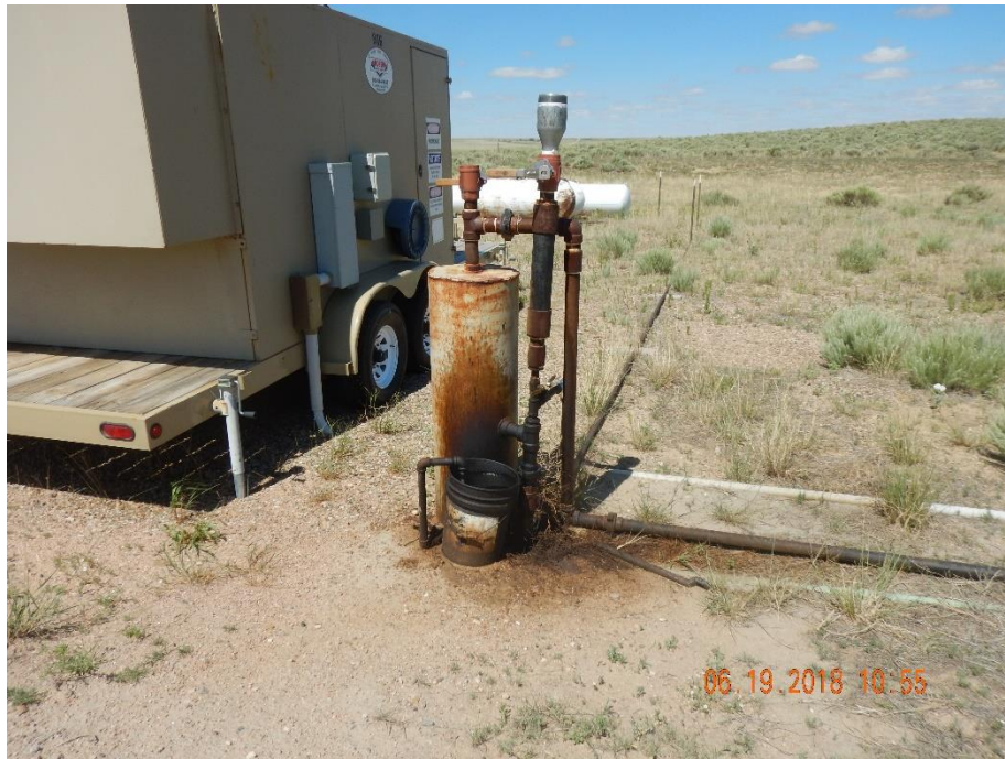
Photo 7: Photo taken from the west end of the location. Photo shows 5 gallon bucket being used to collect chemicals from equipment. Photo also shows stained soils at base. Equipment needs to be repaired to prevent leaks, bucket needs to be removed and properly disposed or placed in containment.
