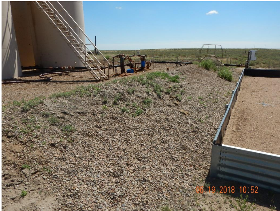
Photo 3: Photo taken from the south end of the tank battery berm, facing east. Photo shows vegetation establishment on the berm. Vegetation compromises the integrity of the containment berms and needs to be removed.
