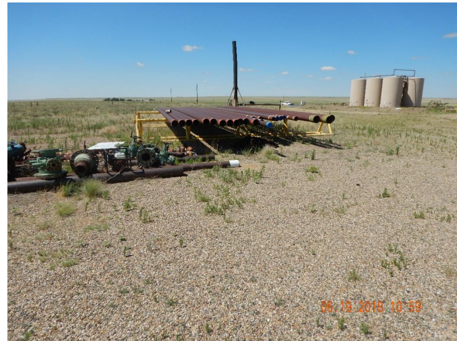
Photo 20: Photo taken from the east end of the location, facing southwest. Photo shows various unused equipment not needed for production being stored on location. This needs to be removed. Additionally, these areas do not appear to be reasonably needed for production and needs to be reclaimed.
