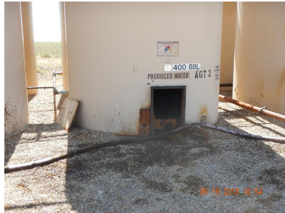
Photo 6: Photo taken from the west end of the tank battery. Photo shows that the manway cover has been removed from the tank. Photo also shows stained soils within berm.
