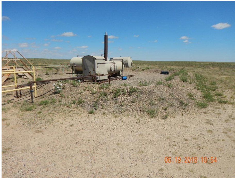
Photo 5: Photo taken from the north end of the location, facing north. Photo shows vegetation establishment on the berm. Vegetation compromises the integrity of the containment berms and needs to be removed.
