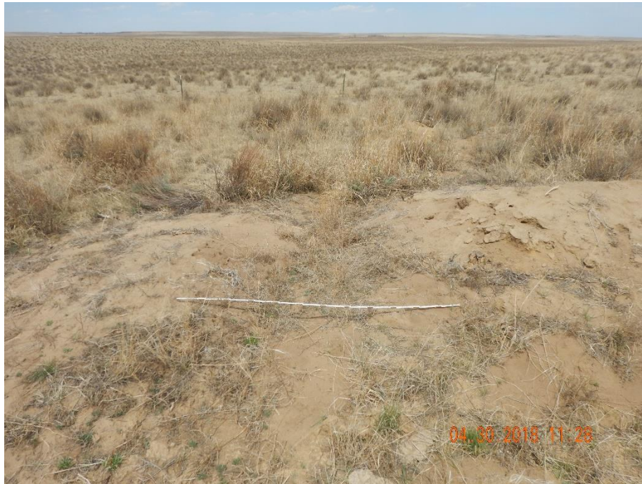
Photo 31: Photo taken from the perimeter stormwater berm on the west end of the location, facing northwest. Photo shows berm is no longer in proper functioning condition, and has “blown out” in this area.
