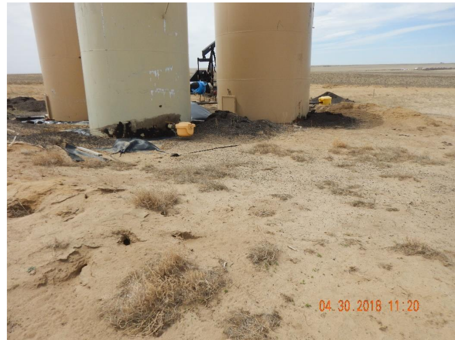
Photo 12: Photo taken from the north end of the tanks on location, facing southwest. Previous inspections documented that the berms around the tanks were inadequate and required operator to repair or install berms, or other secondary containment devices. Photo shows berms, or other secondary containment devices have not been repaired or installed. Photo also shows incomplete signage on the tanks, including NFPA diamond labeling.
