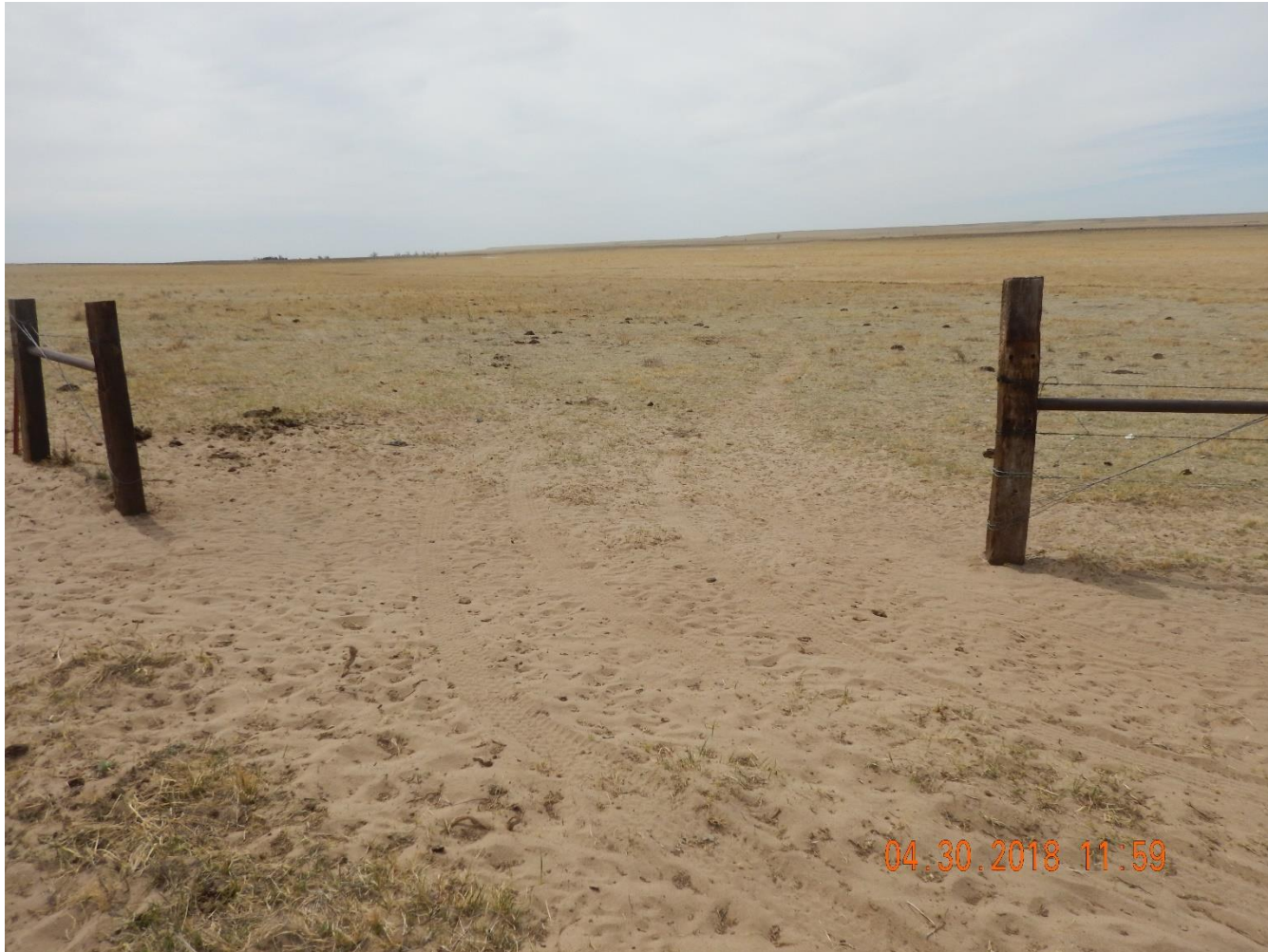
Photo 39: Photo shows gate to the east of the access road. A fence has been constructed across the access road forcing vehicle traffic to drive off road and through this gate in order to access location.
