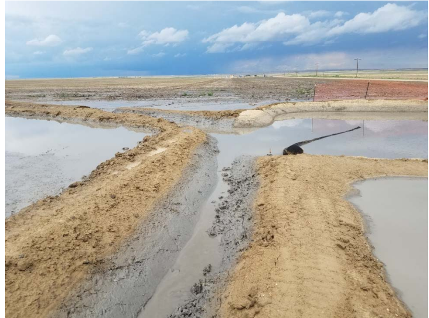
Photo 4 – At the northwest end of the Krier 4 Land Application Area. Stormwater ditches lead to a stormwater detention pond.
