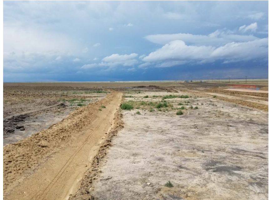
Photo 2 – From north end of Krier 4 Land Application Area at Carlson 22-1 tank battery looking west. Ditches have been cut on the north end of the land application area to aid in stormwater control.
