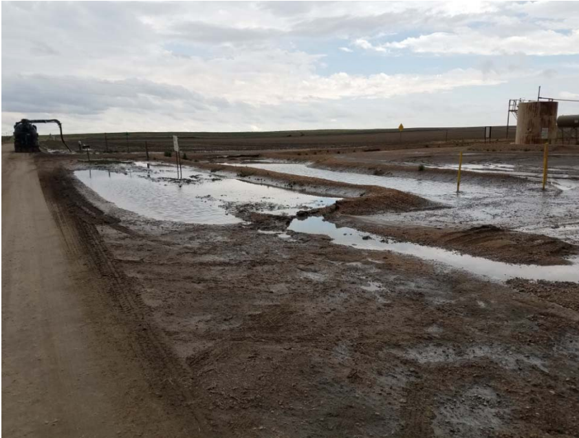
Photo 5 – At DCP compressor station on County Road 68 and 91. Looking east at vacuum truck performing liquid recovery.
