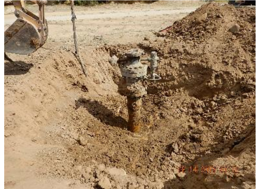
Photo 2: Excavation around wellhead.
