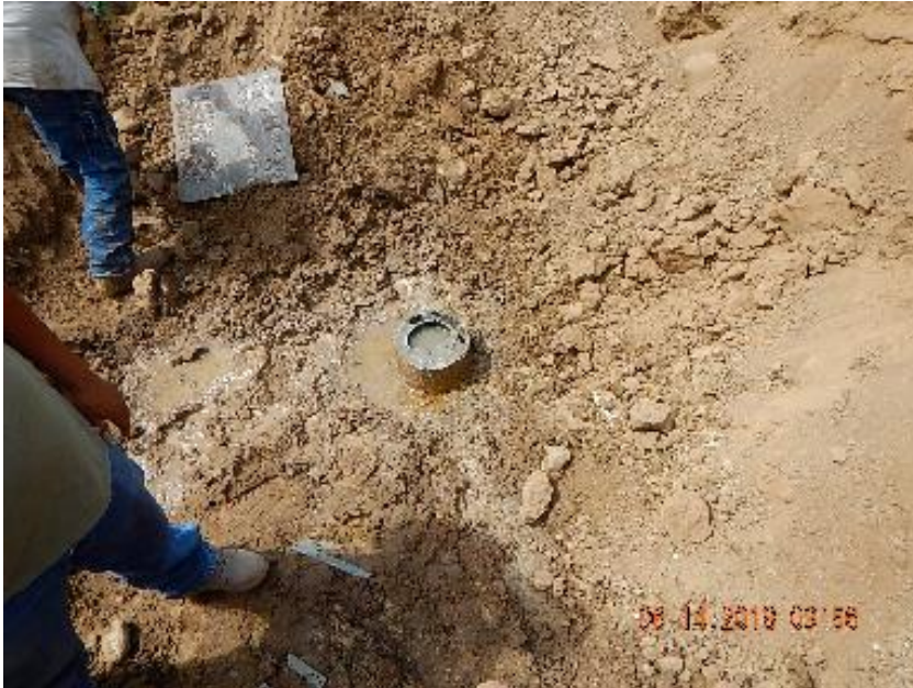
Photo 3: Wellhead cut off and casing with cement to surface.
