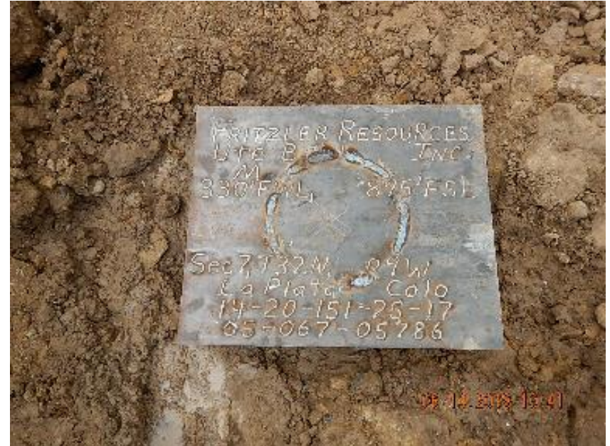
Photo 4: Below grade marker welded to casing.
