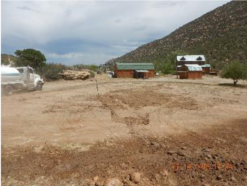
Photo 5: Backfilled excavation with steel riser visible and water truck wetting down site for dust control.
